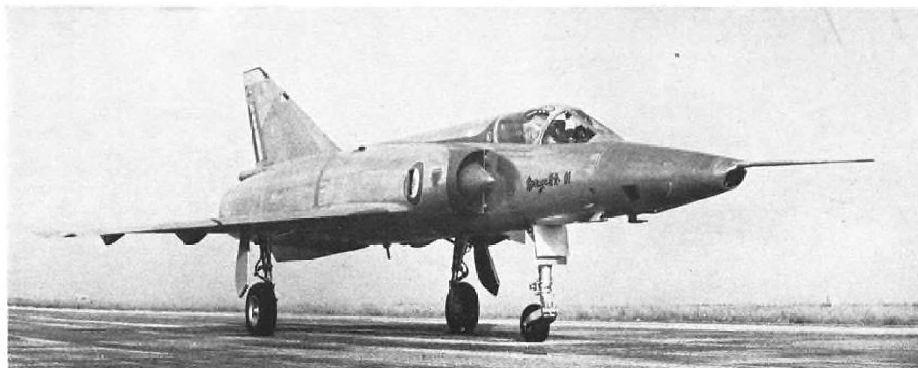
Mirage 3-R reconnaissance model, of which two prototypes are flying, has nose camera installations, one beneath nose probe and another further back on nose. French air force has ordered this version of the Mirage 3 in limited quantities.
