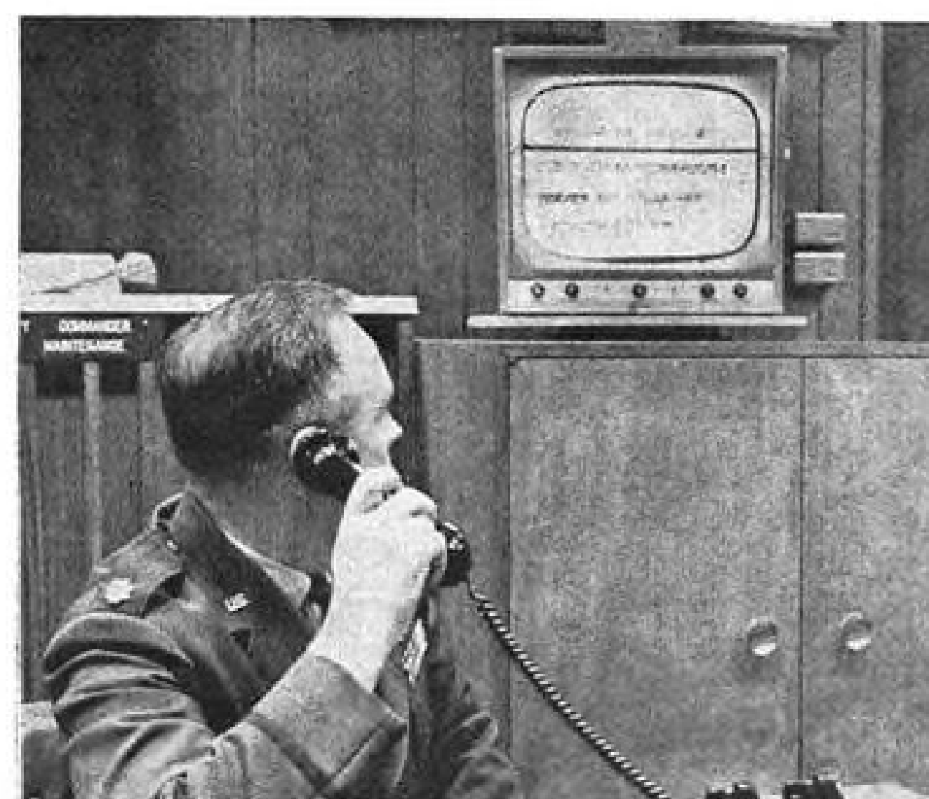
CLOSED CIRCUIT TELEVISION MONITOR in Westover AFB command post provides data for control officers. Seven monitors are located about the installation. Operator's console, right, allows AN/FMQ-5 Automatic Weather Station operators to manually inject data into processing sequence. Other information is received from automatic sensors.
