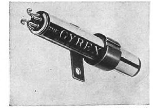
temperature range from —55C to 100C. Dimensions are § in. dia. x 2§ in. long. Device is hermetically sealed. Manufacturer: Gyrex Corp., 3003 Pennsylvania Ave., Santa Monica, Calif.
