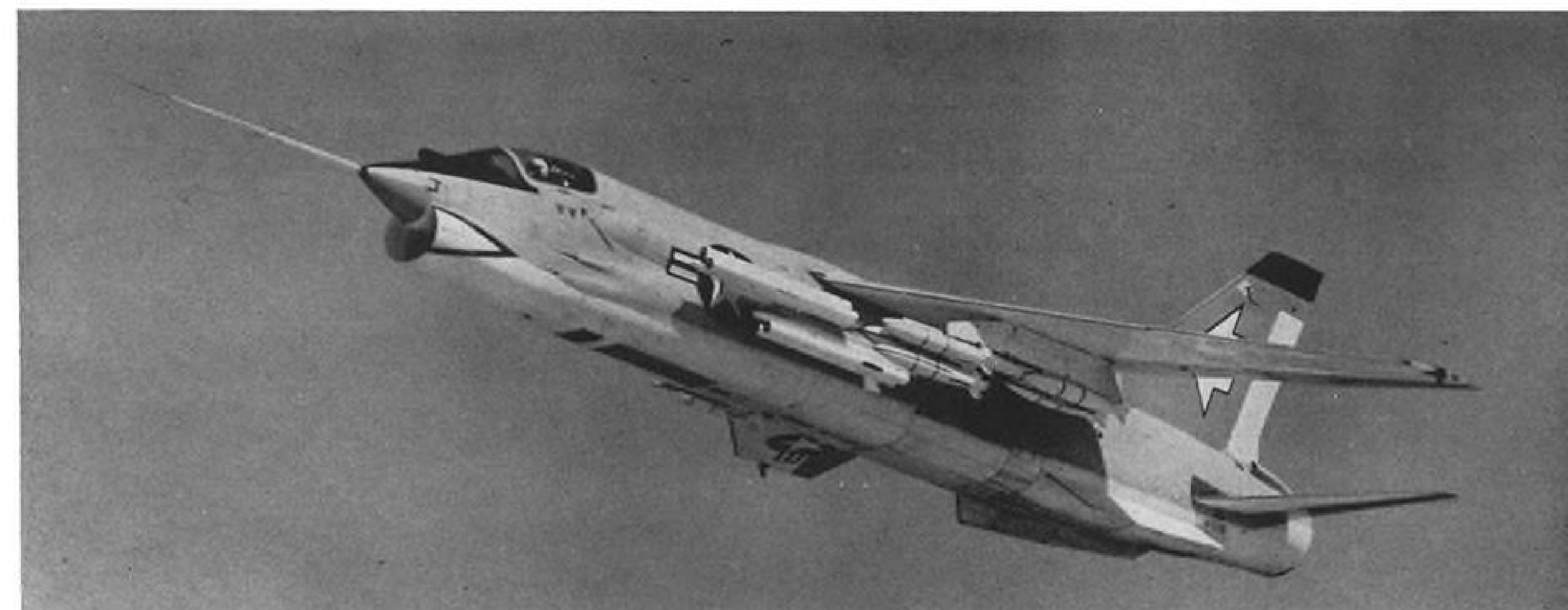
F8U-2NE is airborne with 10 500-lb. bombs on underwing pylons and eight Zuni rockets in fuselage launchers. Other armament carried during evaluation missions included four 20-mm. cannons for aerial combat and low-level strafing runs.
