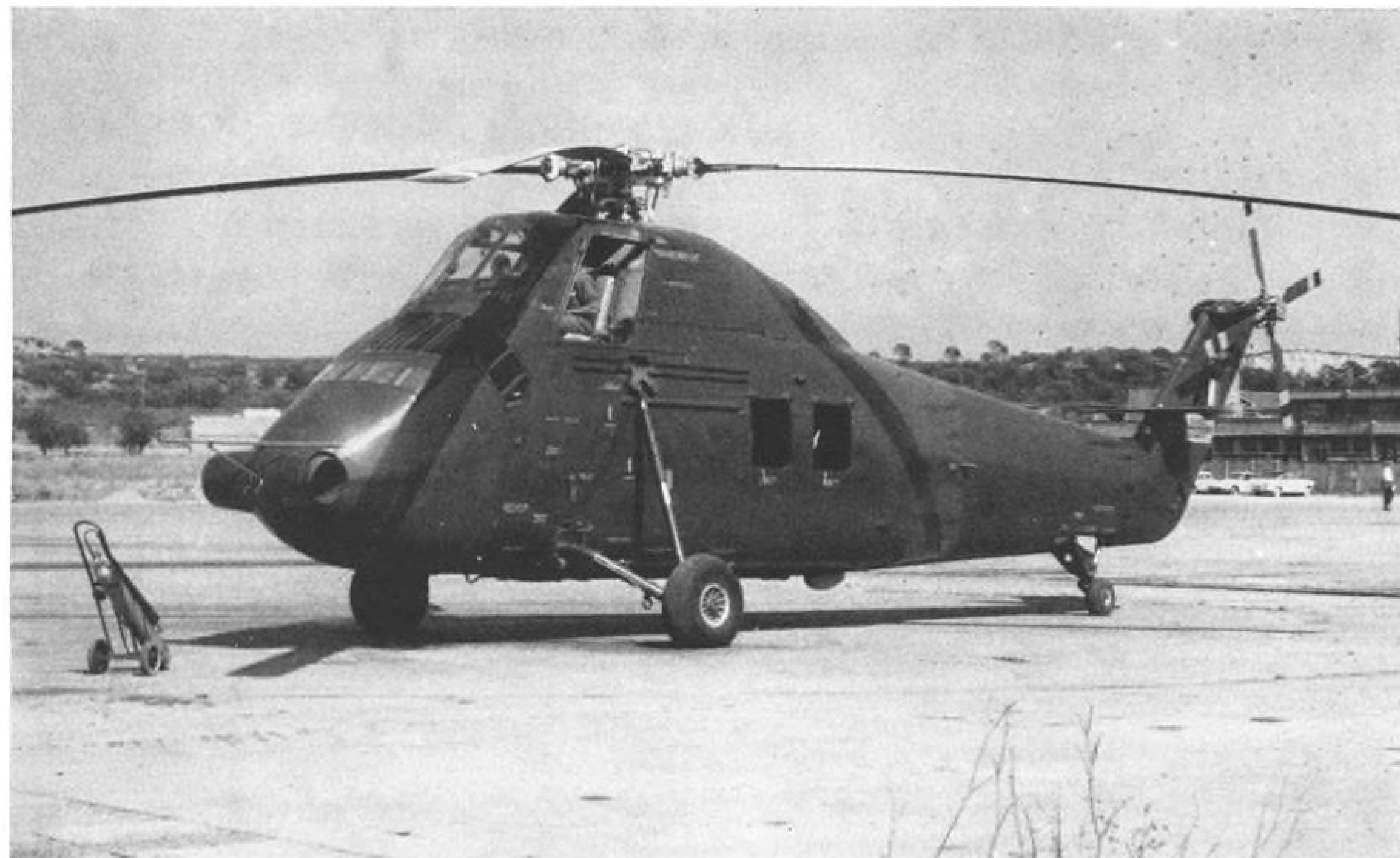
Sud Aviation of France is flying an H-34 conversion powered by paired Turbomeca Bastan turbine engines developing 950 hp. each. Turbomeca is offering the twin Bastan power installation as a retrofit program for the H-34.
