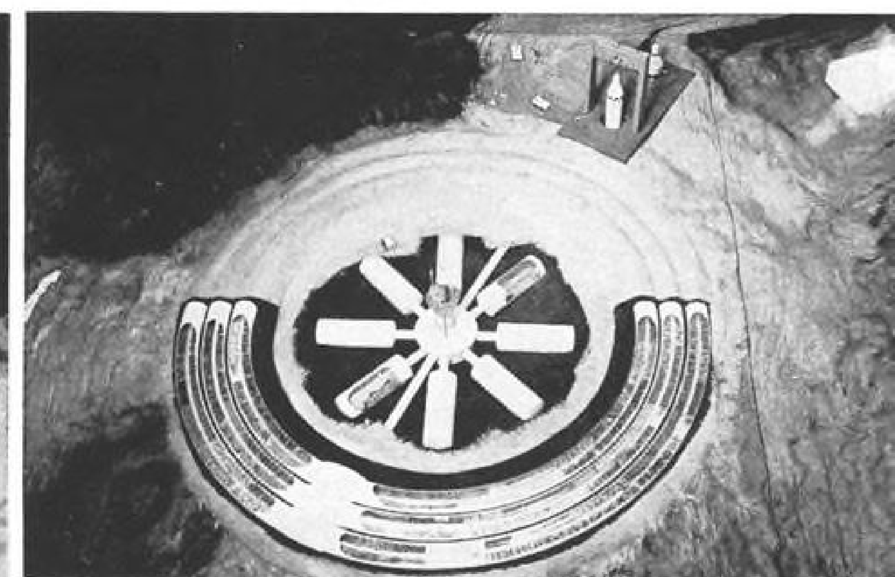
DOUGLAS-PROPOSED SHELTER (left) is covered with lunar soil moved by robot vehicle to give protection against environmental extremes. Operations would be controlled from earth by television and telemetry; TV camera is mounted on vehicle. North American lunar housing concept (right) has underground life center made of clustered booster tanks. Outer rings are closed ecological farm system and for food production, also contain carbon dioxide-to-oxygen converters and depository for biological byproducts.
