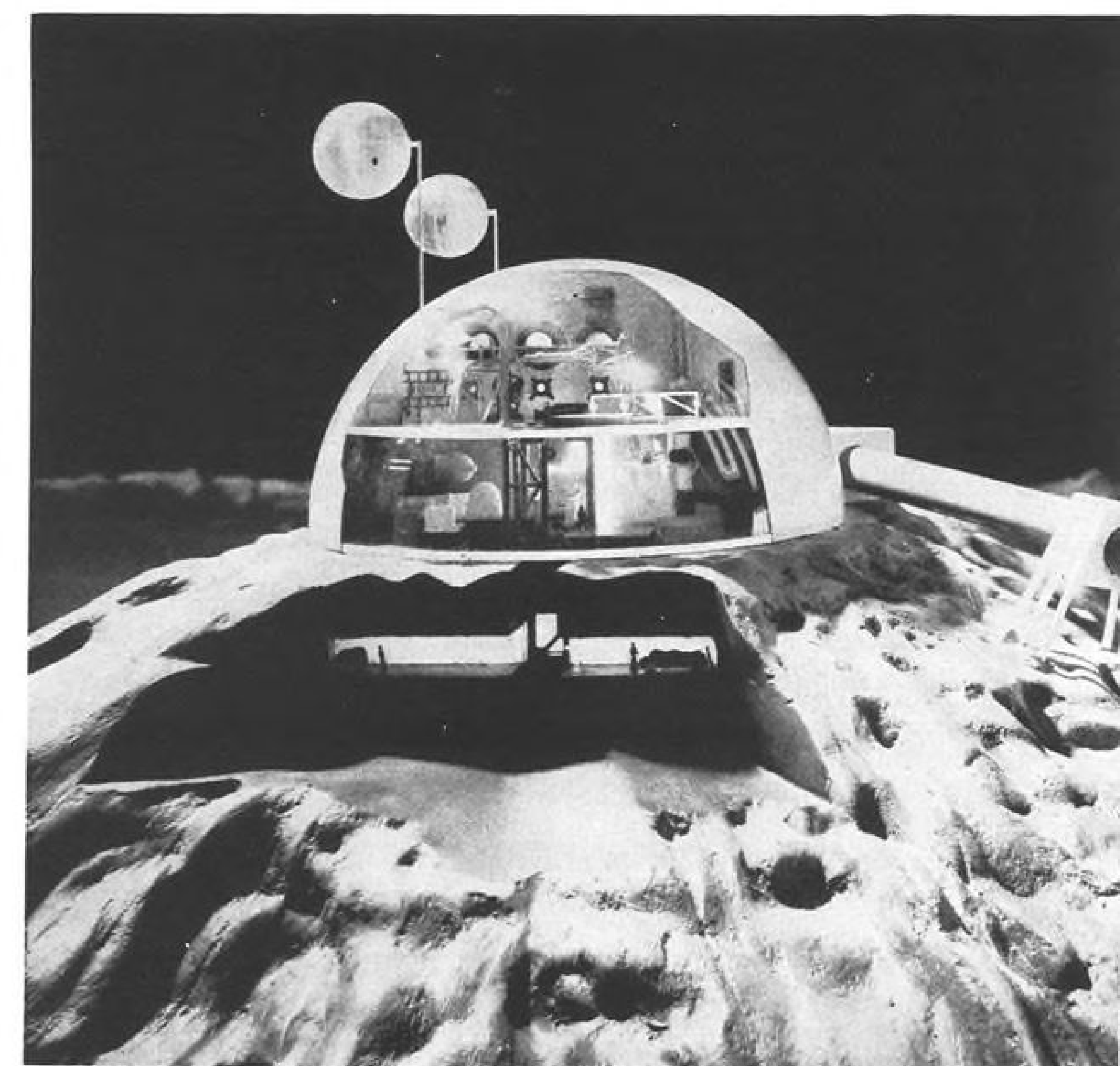
WATER-CONVERSION PLANT is modeled in North American Aviation concept. Cupola covers a fissure from which volcanic rock has been removed and processed to furnish water by crushing the rock and then heating it. Rock residue can be used for construction purposes after water has been removed.
