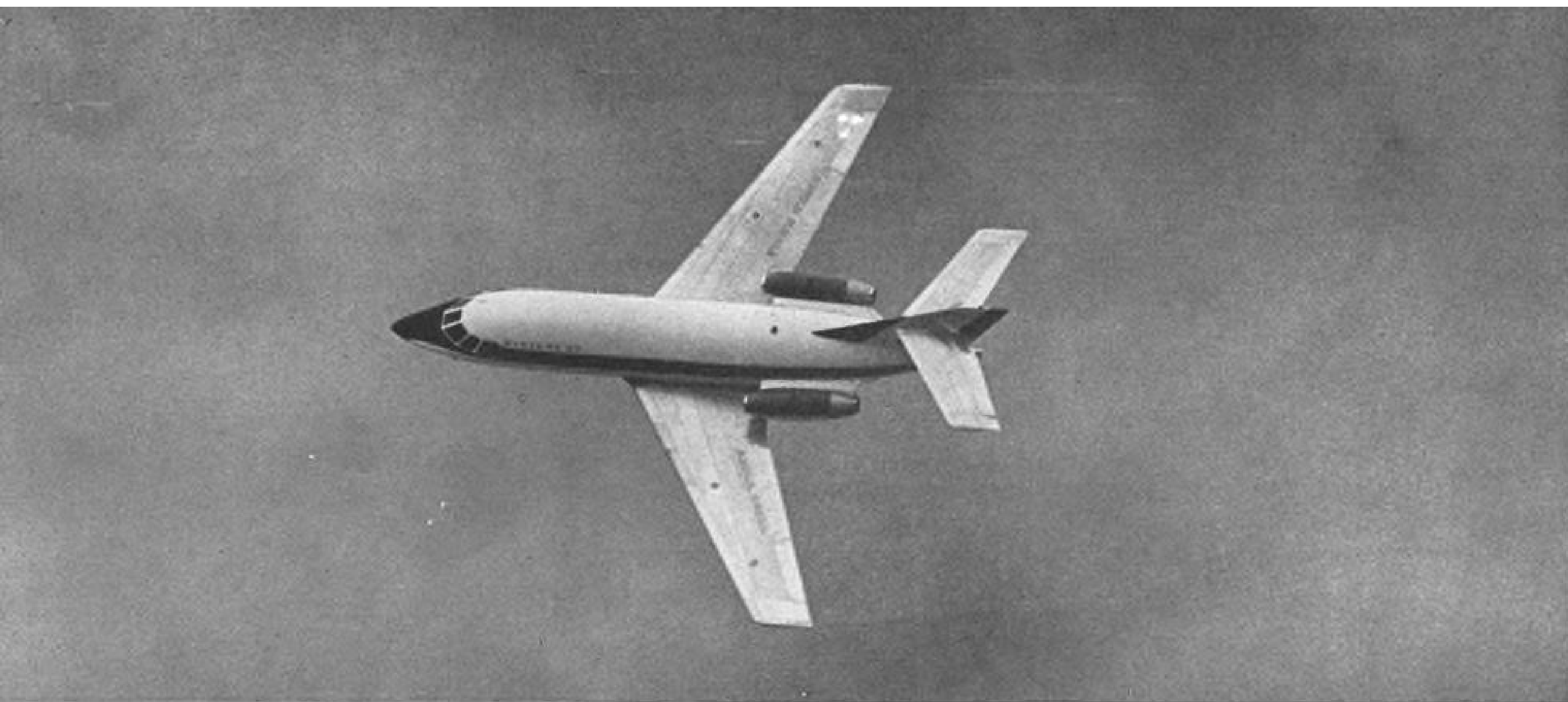
Dassault Mystere 20, powered by Pratt & Whitney JT12A-8s in eight-passenger configuration, has maximum takeoff weight of 19,290 lb.
