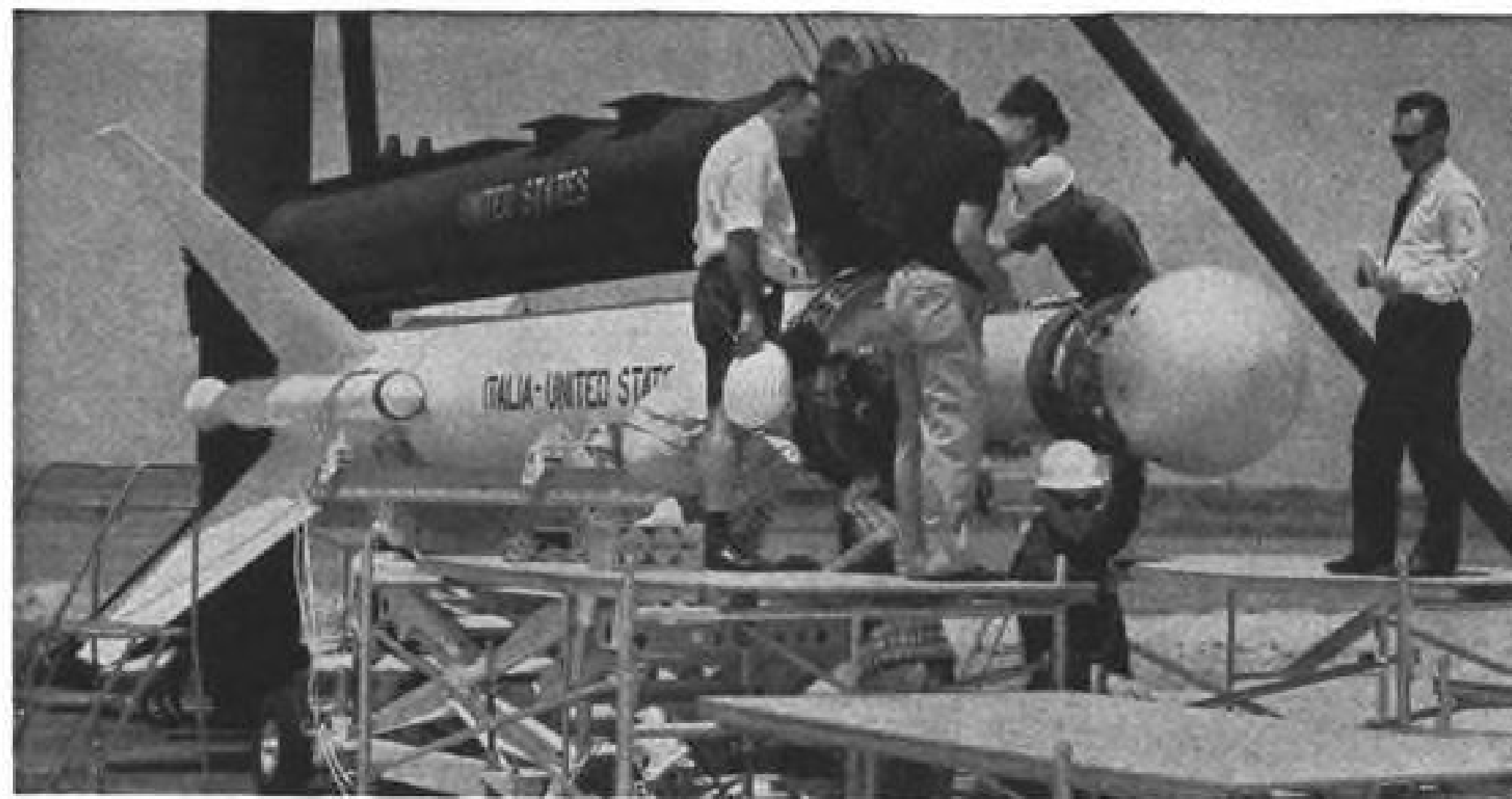
SAN MARCO PAYLOAD is prepared for a sounding rocket test from Wallops Island, Va., by U.S. and Italian technicians. The payload is shown both with the fairing removed and in place. San Marco, which is scheduled to be launched from a platform in the Indian Ocean near the equator, is one of a number of bilateral space projects in which the U.S. is involved. The sounding rocket, called Shotput, consists of a Thiokol Pollux E6 first stage with two Thiokol Recruit assist rockets. At launch, the combination provides 120,000 lb. thrust. The second stage is an X248 Altair, manufactured by Hercules Powder Co.-Allegany Ballistics laboratory. The vehicle has a launch weight of 11,000 lb., and is 32 ft. long with a 33-in. dia.
