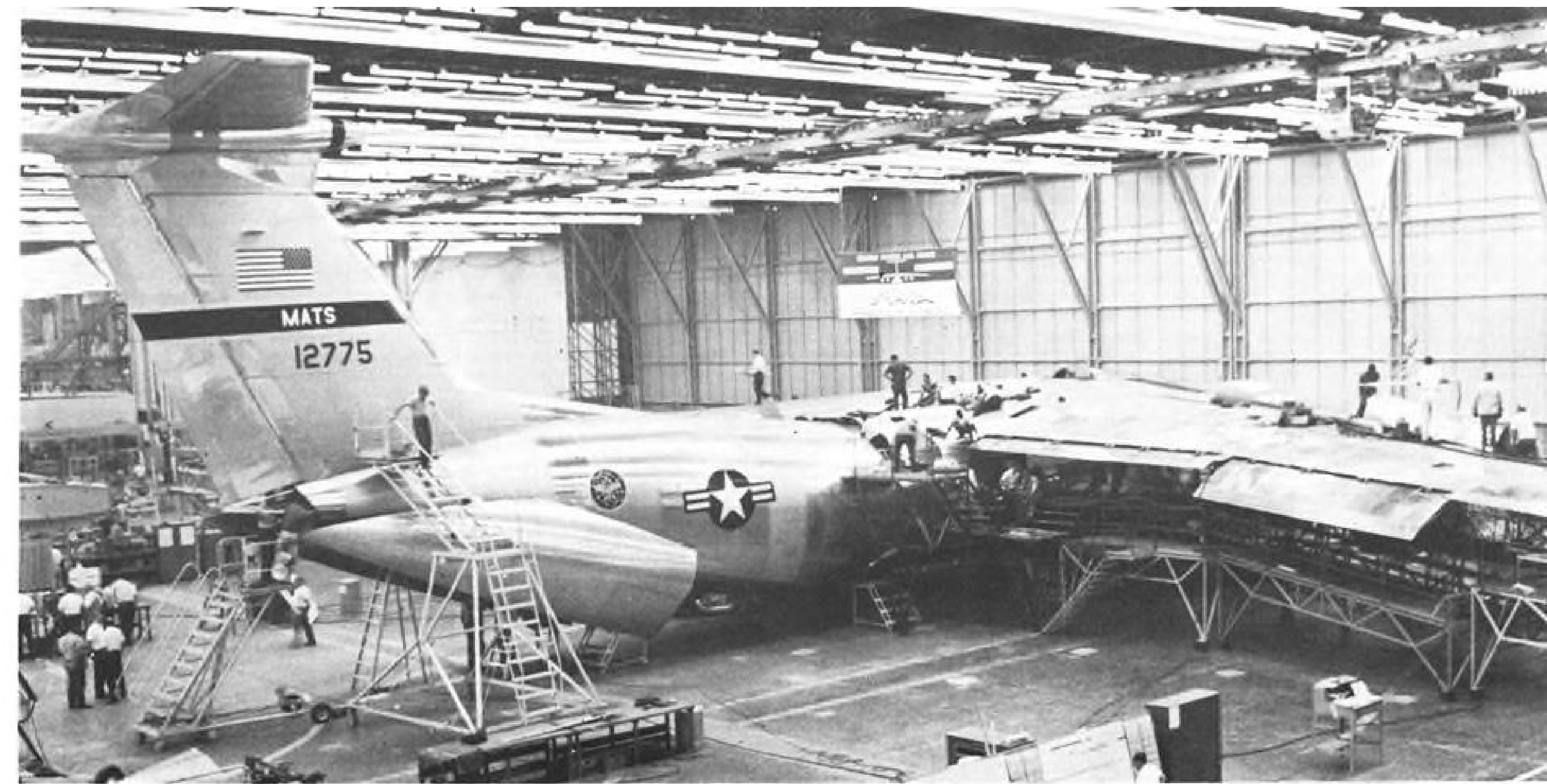
FOWLER FLAPS are the only high-lift devices on the C-141 wing. Horizontal stabilizer trim axis is 12½ deg. down and 4 deg. up.
