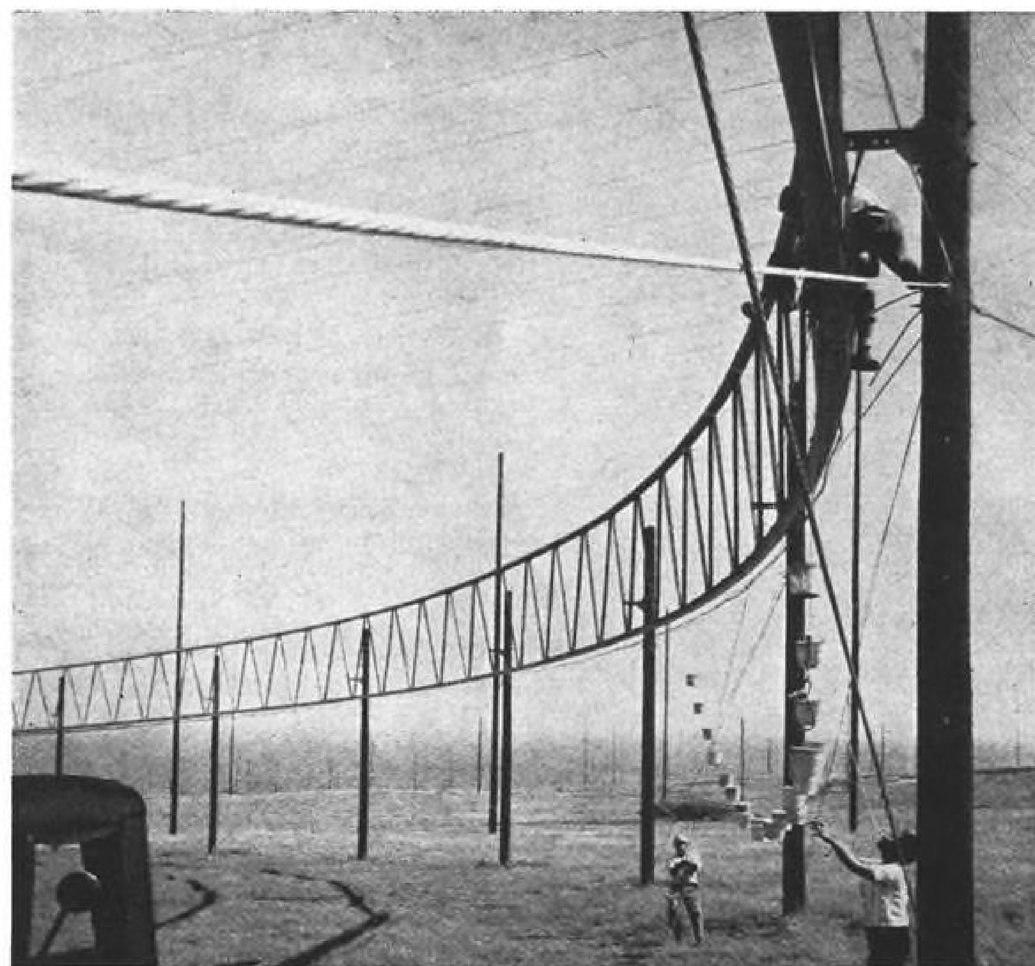
WEIGHTS ARE ATTACHED to wires of the horn surface strung over the ring truss to create proper tension before the wires are attached to the upper truss ring. Area between truss and outer perimeter of poles is bridged by wires comprising horn upper surface.
