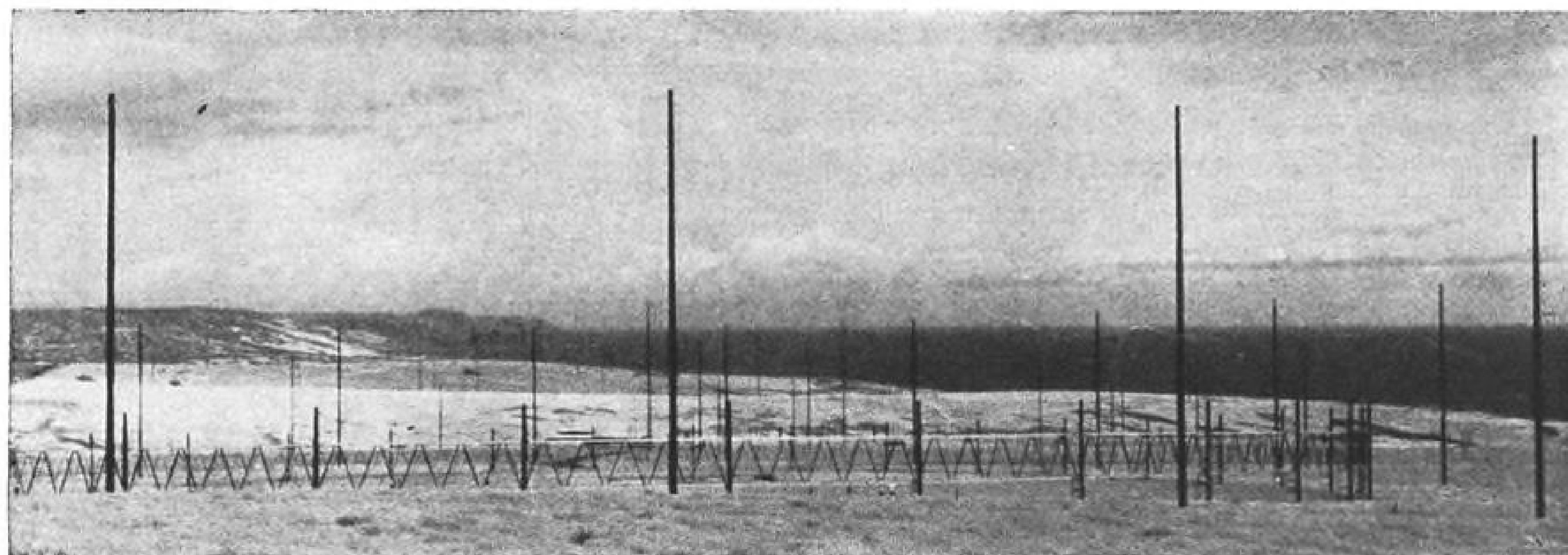
WIRE GRID HIGH FREQUENCY Luneburg lens antenna being built by TRG-West at Molokai Island, Hawaii, for the Federal Aviation Agency is expected to lead to improved HF air-to-ground communications and large savings in land area required by ground antenna systems. Ring truss, which supports double wire grids of the lens, is assembled on the ground before being hoisted onto vertical poles.
