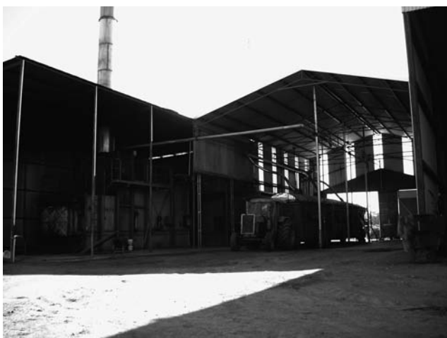
FIGURE 4.22 Distillation plant with container technique.
