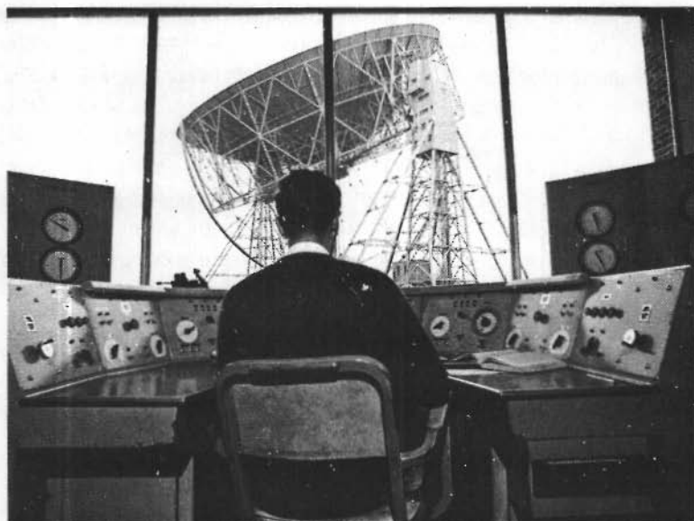
FIGURE 12-2. The giant 250-foot diameter radio telescope at Jodrell Bank, Cheshire, England. The world's first really big radio telescope, it is still (1970) the largest that can be steered to point anywhere in the sky. This photograph was taken from inside the telescope's control room. Courtesy of the Ronan Picture Library.
