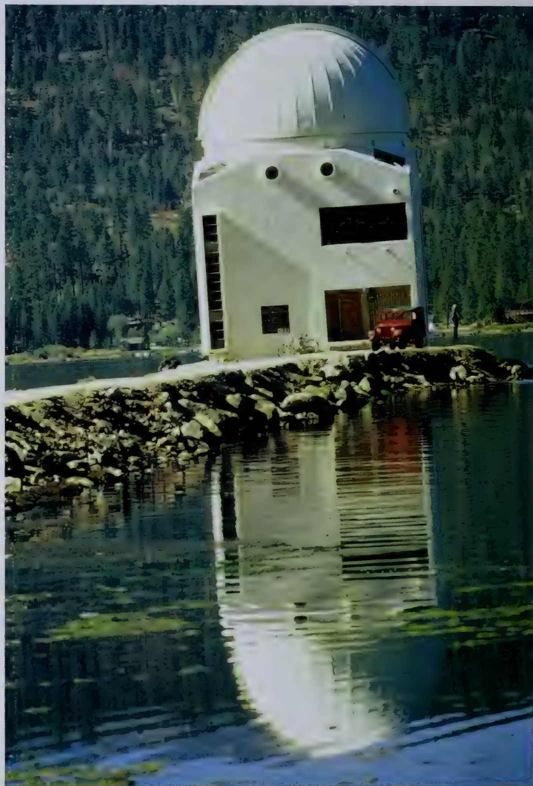
6.6 Big Bear Solar Observatory stands in the middle of a lake because studies have shown that the earth's atmosphere is calmer above bodies of water than above land.
