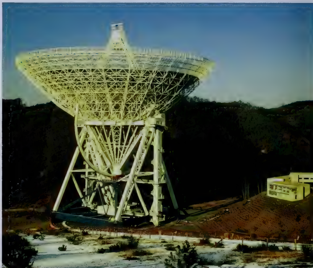
8.14 Great radio telescopes, such as this one at Bonn, West Germany, are used around the world to gather and record radio emissions of celestial objects. The diameter of this dish is 100 meters, more than a football field across.
