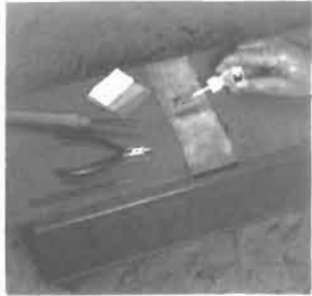
4. Applying the adhesive
