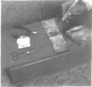
8. Soldering and fixing the cables
