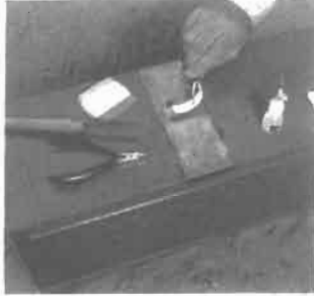
5. Spreading the adhesive
