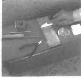
2. Cleaning of the application area
