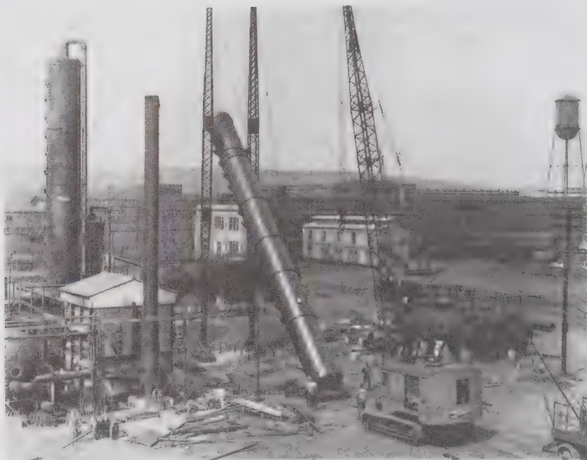
Installation of distillation columns for coal-tar products at Bound Brook, 1935. (Edelstein Library.)
