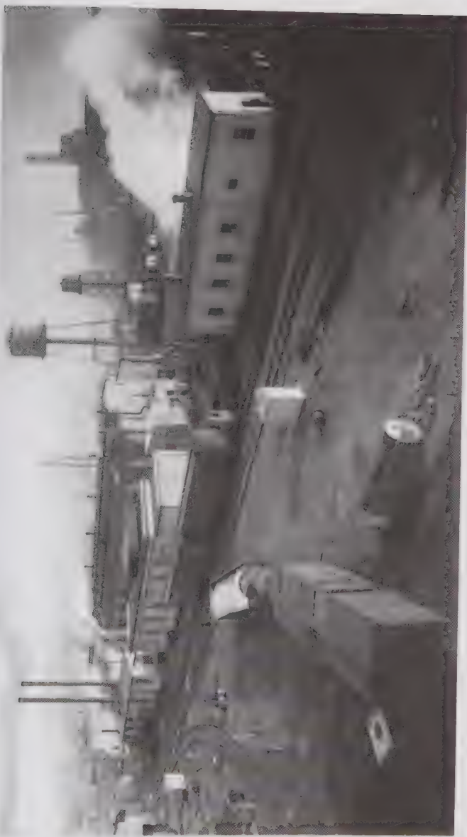
Calco Chemical Company, around 1917. View looking north, showing the then largest building, no. 8 (later no. 30), where beta-naphthol, azo dyes, and dimethylaniline were manufactured. In front are, from left to right: building 11, the refrigeration plant; building 9, the boiler house; and the transformer house. Buildings 1, 2, and 3 are behind building 8. In the right distance is the Hemingway & Co. insecticide factory. Note the extent of rail sidings at this time, the barrels in which products such as beta-naphthol were distributed, the boundary fence separating the "West Works" from the "East Works," and the water tank marked "Calco Chemical Co." To the north is the Central of New Jersey Railroad, and, beyond, the Heights of Middlebrook. The three-story administration building was located to the left of the area shown. (Edeistein Library.)
