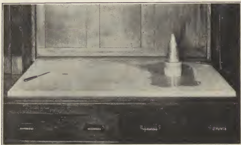
FIGURE 1.—MULLER AND SLAB, SHOWING METHOD OF RUBBING OUT COLORS.
