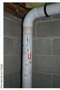
The white pipe in these photos is part of an Active Soil Depressurization system to mitigate radon in a New Jersey home. The U-tube manometer liquid level differential in the photo indicates that the exhaust pump is functioning properly.
