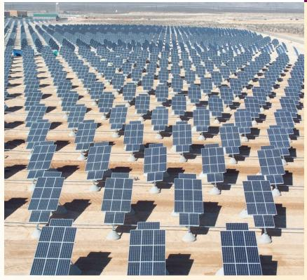
Nellis Air Force Base in Nevada has a giant solar panel power array that generates about 14 megawatts of power for the base. This provides about 25% of the electrical power needs for the base.
