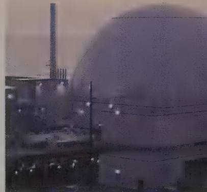
Containment shell around nuclear reactor.
