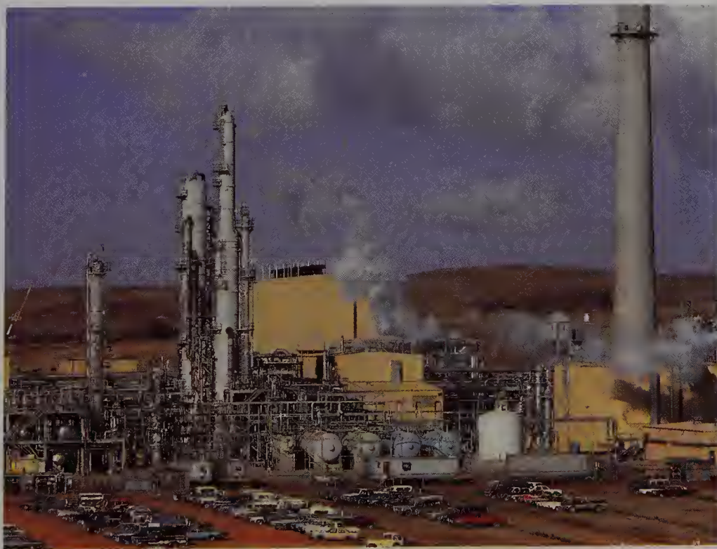
Figure 5-4 Tenneco's Great Plains coal gasification plant in North Dakota, where coal is converted into a combustible gaseous mixture, as in the water-gas reaction. This plant is able to produce over 400 million liters of combustible gas per day.
