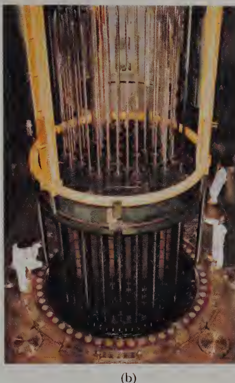
Figure 21-11 Diagram of the core of a nuclear reactor. (a) The fuel rods contain the fissionable material. The control rods consist of a material that is a good absorber of neutrons. By raising and lowering the control rods, the density of neutrons in the core, and thus the rate of production of energy, can be controlled. (b) Loading of fuel rods into a nuclear reactor core. The fuel rods are the long, thin, shiny metal tubes, which are filled with fissionable material.
