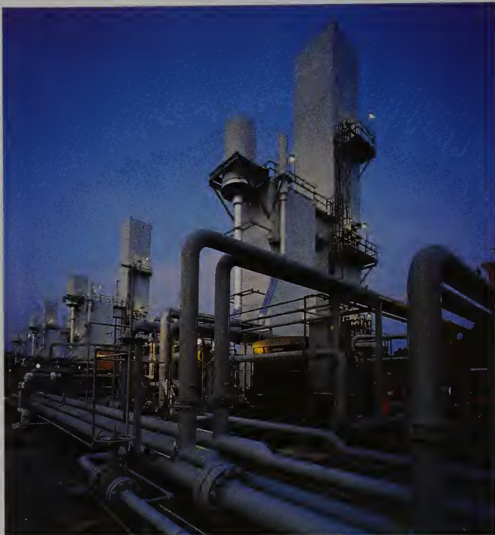
A nitrogen production plant at Jay Field in western Florida. The nitrogen is obtained by the fractional distillation of liquid air.
