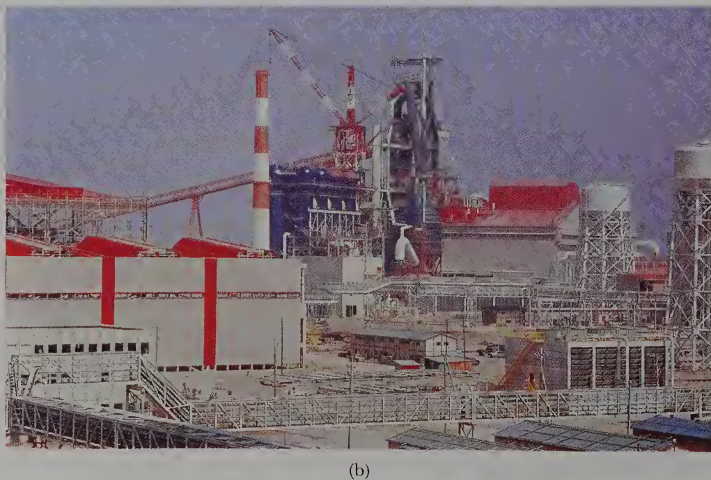
Figure N-7 Iron is produced in a blast furnace. (a) A diagram of a blast furnace. (b) A typical blast furnace like the one shown here runs continuously and consumes about 120 railroad cars of iron ore, 50 railroad cars of coke, and 40 railroad cars of limestone per day. The 5000 tons of iron produced requires about 75 railroad cars to transport it.
