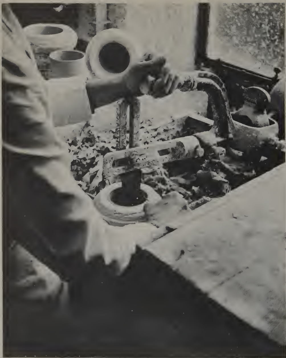
XXVI. Cup making with the lever jolley
