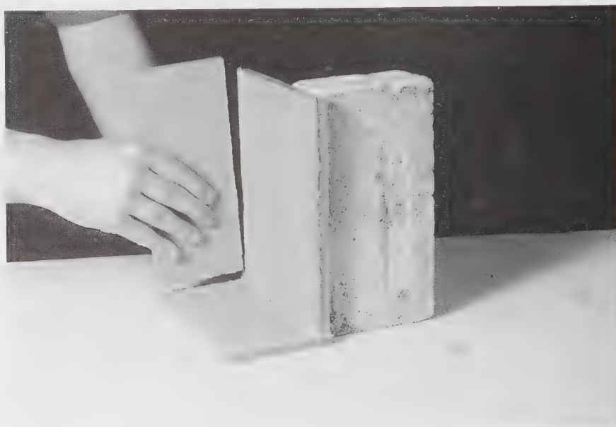
6-60 As the slabs are assembled, props like this brick may be needed to hold the slabs temporarily in place.
