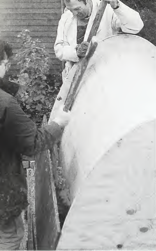
Jack compacting castable for kiln arch.
