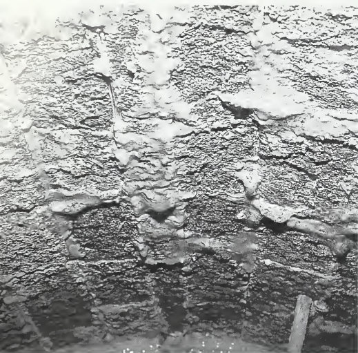
A crust forms on the walls of my soda kiln made of HT1 bricks.
