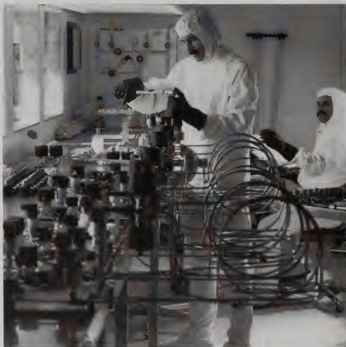
Figure 7.7.2. Connection work in a high-purity room. Courtesy of the Messer Group, Frankfurt-am-Main, Germany.
