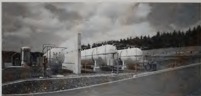
Figure 5.2.11. Hydrogen storage tanks for the solar hydrogen project. Courtesy of Linde AG, Wiesbaden, Germany.
