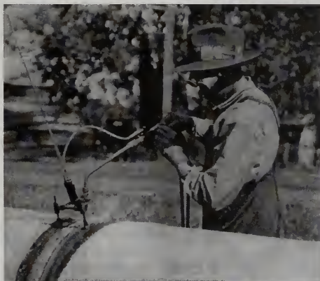
Figure 6.6.7. Oxyacetylene welding on a leaking pipeline.
