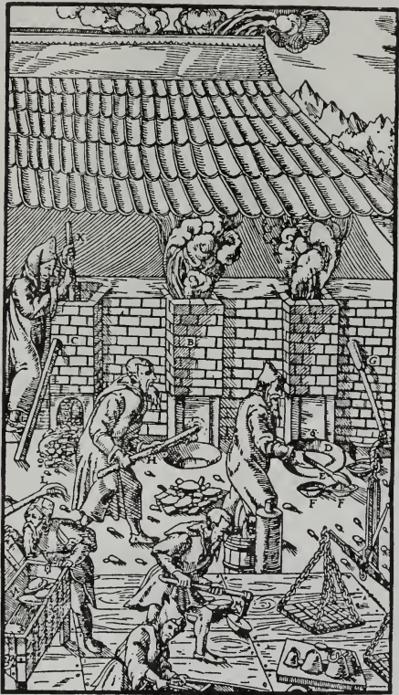
Figure 7.3.1. Blast furnaces for smelting copper–lead ores. From Agricola, De re metallica , 1556.
