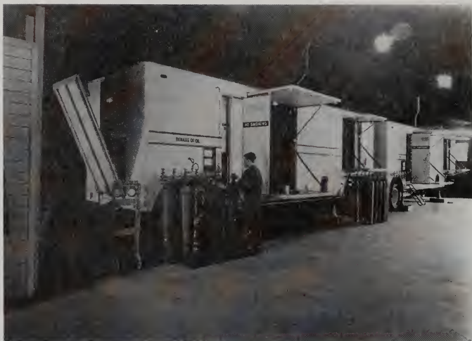
Figure 5.9.2. Mobile oxygen generators being used in Alaska by 1944. From Butrica (1990) with permission.
