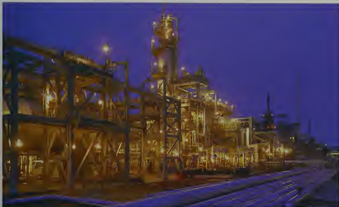
Figure 2.5 Distillation tower used in the refining of crude oil.
