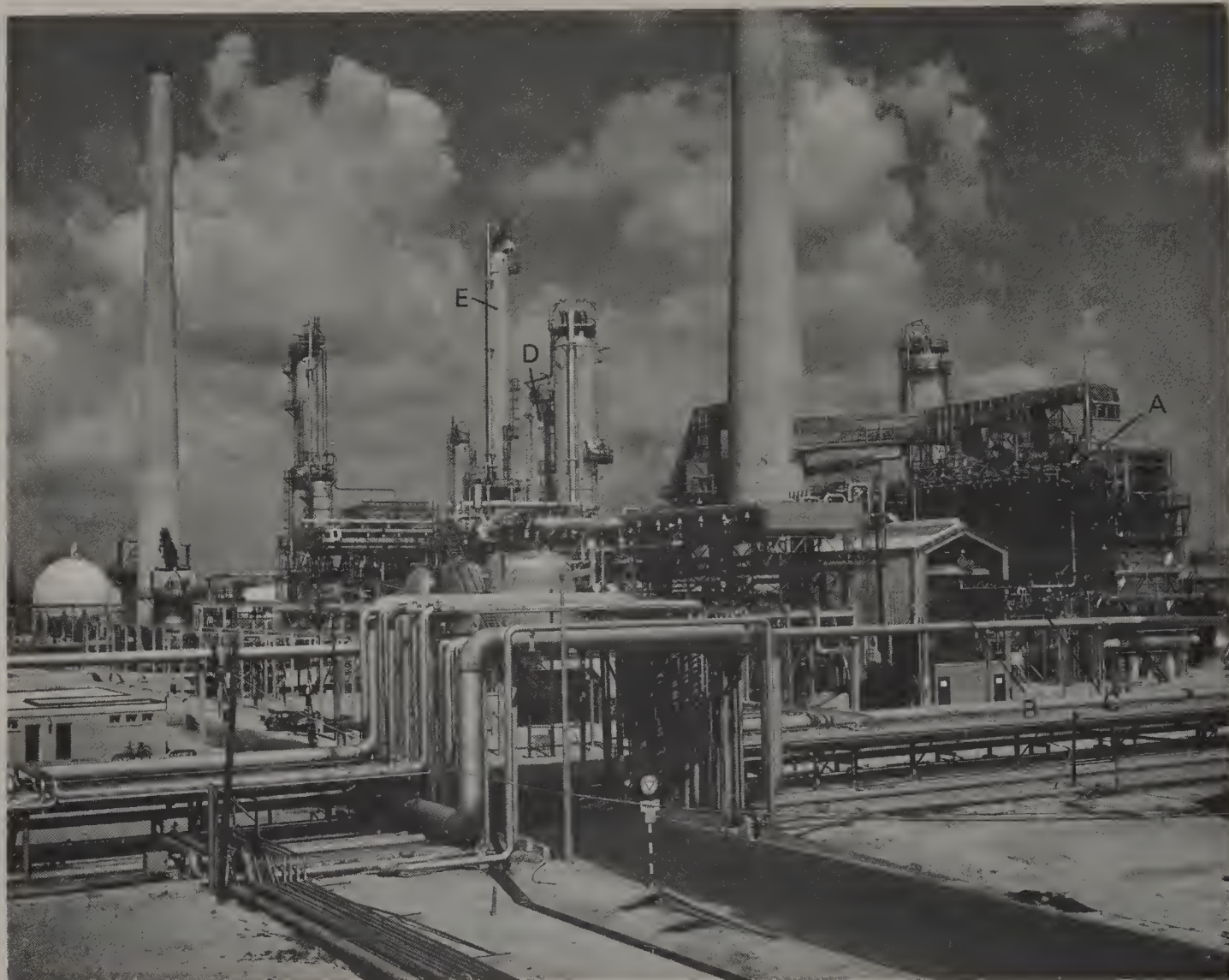
Plate 8.1. A reforming unit. Naphtha is heated in a furnace (A), mixed with hydrogen, compressed to a high pressure (B) and passed over a heated platinum catalyst. The reactors are hidden in the photograph (C). Low boiling hydrocarbons are removed by fractional distillation, for example ethane, propane, butane (D). The residue, which is fractionated (E), contains principally the aromatic hydrocarbons, benzene, methylbenzene and dimethylbenzenes (Esso Petroleum Co. Ltd.)
