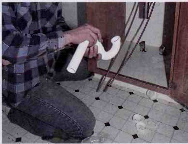
This plumber is installing pipe fittings made of polyvinyl chloride. ( David R. Frazier Photography )
