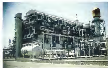
This plant in Tokuyama, Japan, passes ethane rapidly over a hot catalyst. The products are ethylene and hydrogen.
