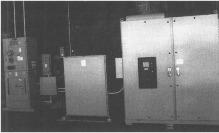
Figure 4.4 300 kW rapid charger for charging electric buses (By courtesy of Norvic, Inc.)
