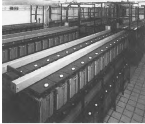
Figure 8.6 Large UPS battery room (By courtesy of Tungstone Batteries Ltd)
