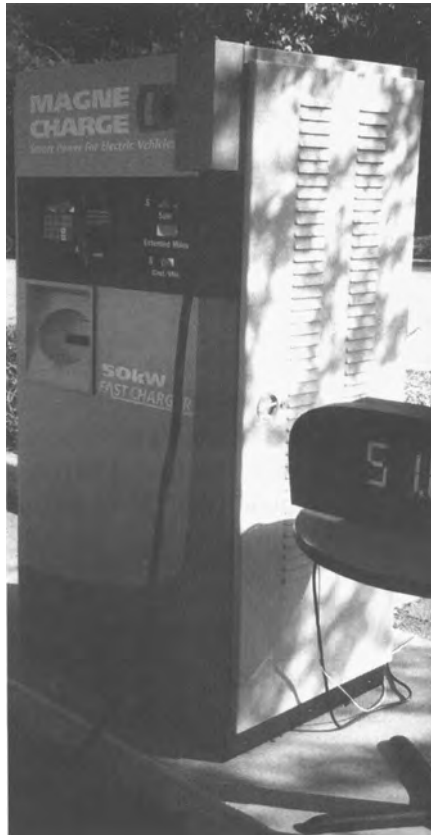
Figure 4.7 Magne-Charge® 50 kW inductive fast charger, as installed in California and Arizona (By courtesy of Batteries International)
