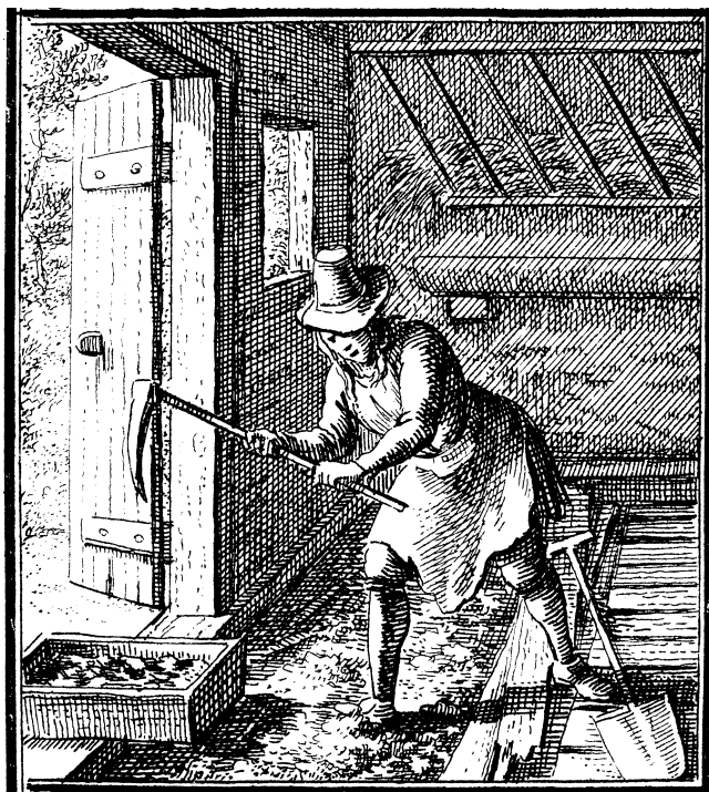
Fig. 37. A saltpetremen at work, pulling up the floor in a stable to get to the earth beneath. An engraving from a broadsheet issued by a Swiss firework manufacturer in the early eighteenth century.
