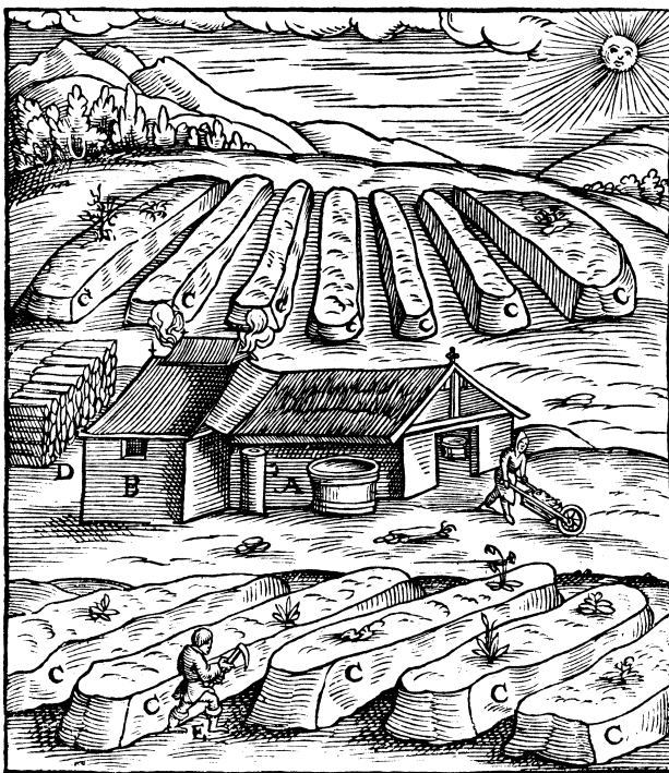
Fig. 38. Artificial nitre pits shown in a woodcut from Ercker's mining work from 1580.
