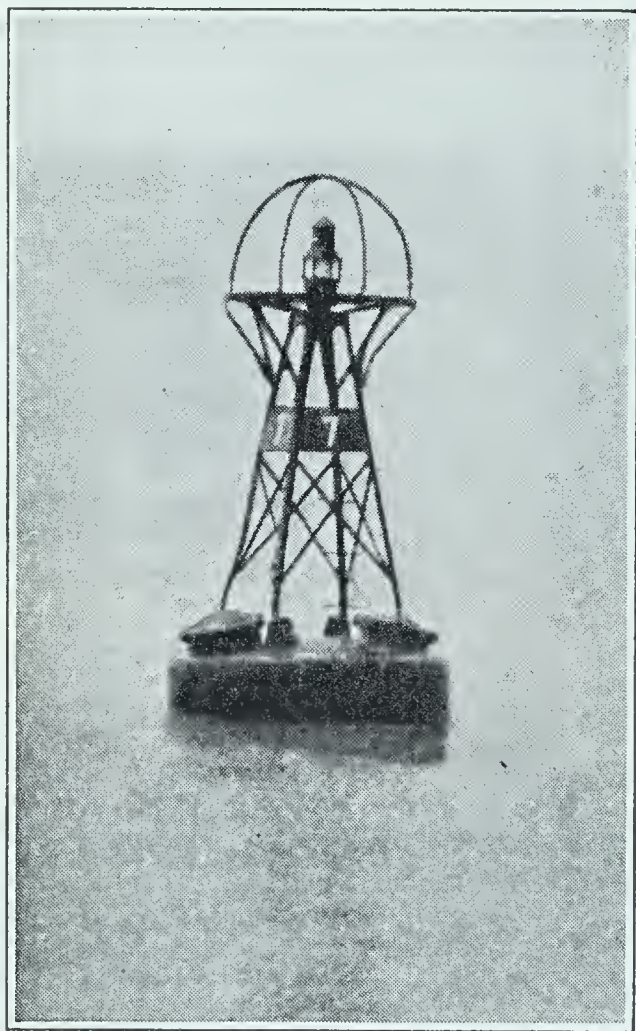
FIG. 316. Buoy lighted with acetylene, for marking ships' channels
