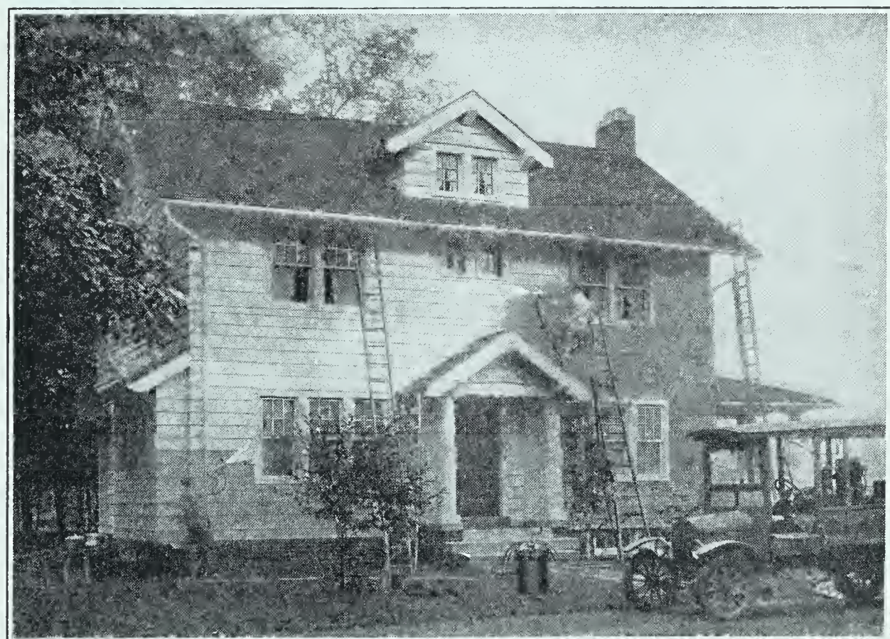
FIG. 404. Spraying a house with white paint containing zinc oxide and lithopone
