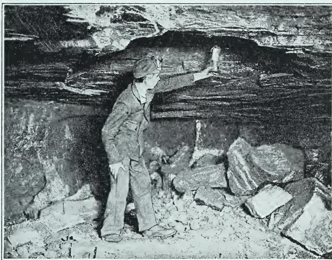
FIG. 331. Testing for pockets of explosive gas mixture in a mine
