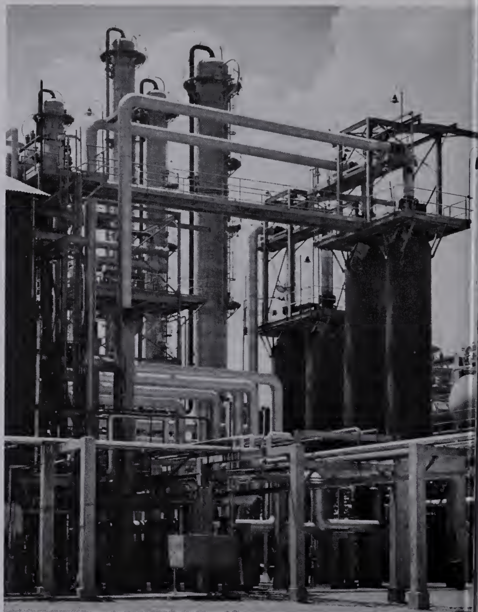
A catalytic reforming unit. Alkanes in the heater on the left go into four reactors (on the right) that contain platinum catalyst. The aromatic molecules produced there go to the tall distillation columns (center, rear) for separation into benzene, xylene, and so on. (Courtesy of the Shell Oil Co.)
