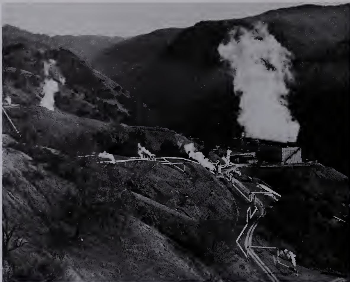
Fig. 4-10 Part of the Geysers power plant in Northern California. Note the steam pipes with expansion loops in the foreground. (Photo courtesy of the Pacific Gas and Electric Co.)
