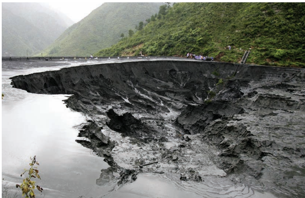
A broken spillway from a vanadium mine in northwest China in 2008 contaminated two nearby rivers with ore tailings. ( Reuters Limited )
