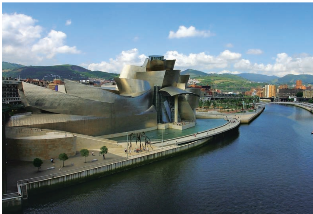
The Bilbao Museum in Spain incorporates highly reflective external titanium panels. ( Cornel Achirei/Shutterstock )
