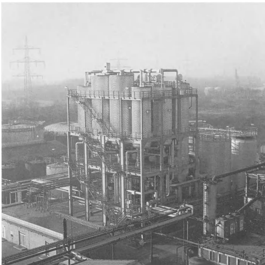
Figure 9.6: Rütgerswerke's crystallization plant at Castrop-Rauxel/West Germany for the production of refined naphthalene
