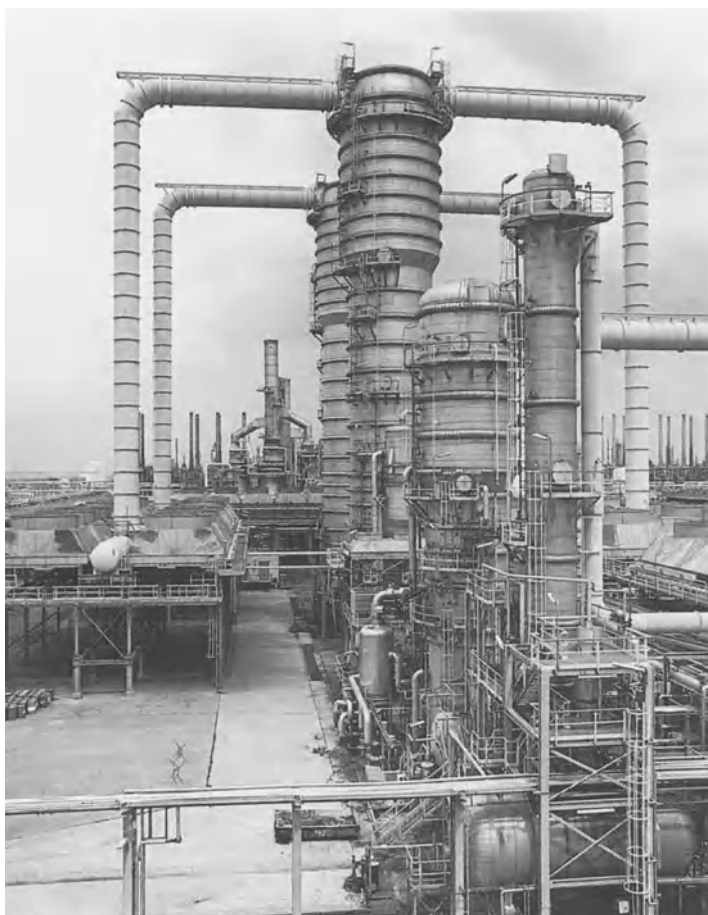
Figure 5.9: Part of the styrene distillation plant operated by Dow , Terneuzen/Netherlands
