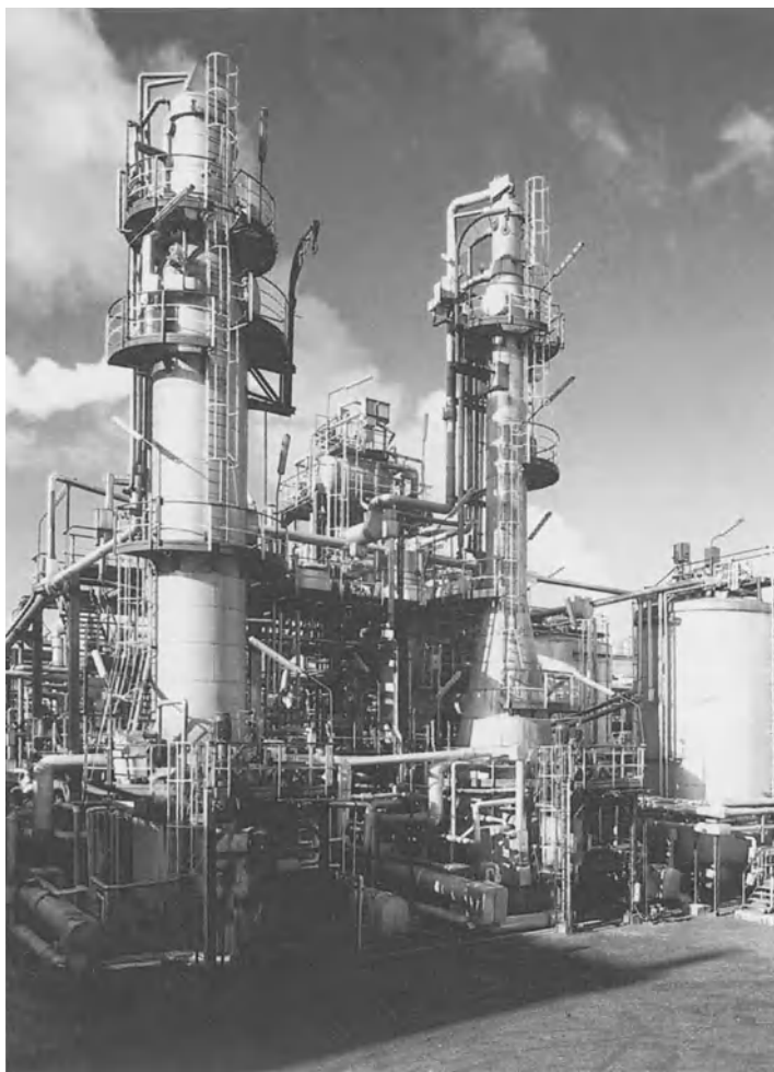
Figure 7.2: Thermal pretreatment and distillation units of the PA plant of Hüls/Veba , Bottrop/West Germany
