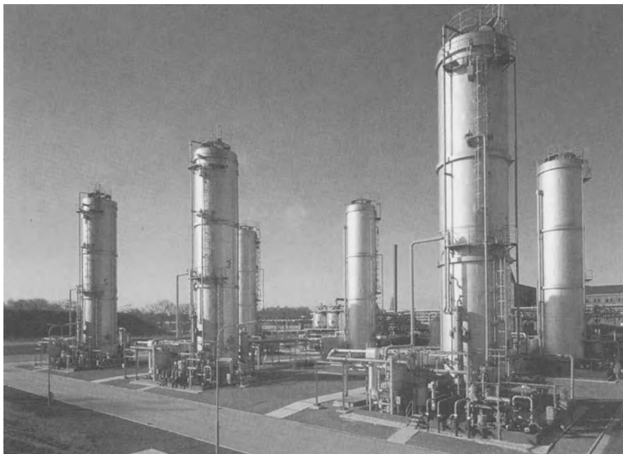
Figure 5.13: Oxidation reactors for the production of phenol from cumene, Phenolchemie , Gladbeck/West Germany
