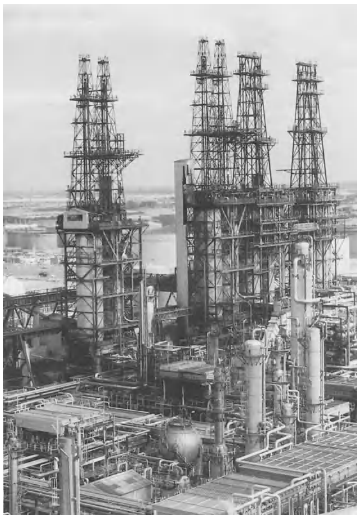
Figure 13.9: Delayed coker operated by Conoco , Immingham/ England
