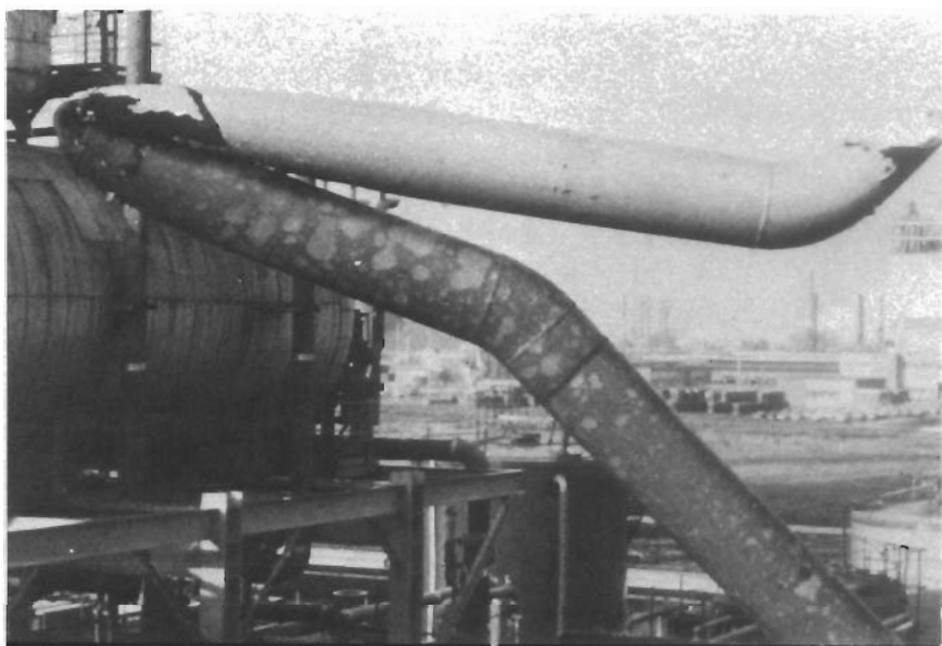
Figure 10-4. This relief-valve tailpipe was not adequately supported.
