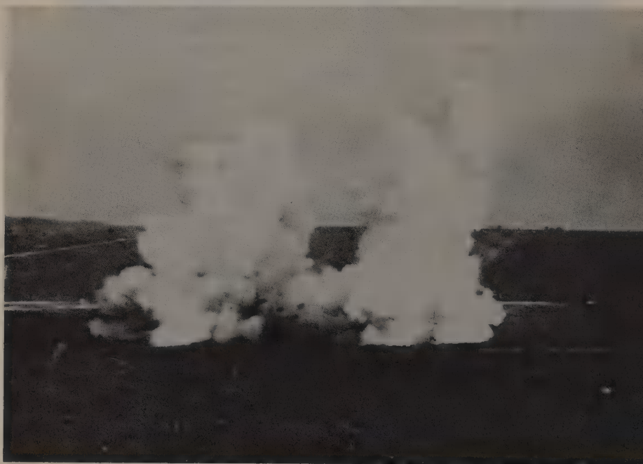
3 & 4 The British chemical weapon which the Germans feared most. Above , Livens Projectors, fired in batteries of 25 at a time; each sent a drum of 30 lbs of liquid phosgene hurtling into the enemy's lines. Below , on impact a burster of TNT releases a dense cloud of gas. At the Battle of Arras in 1917, the British fired over 2,000 Livens bombs simultaneously in one mass attack.
