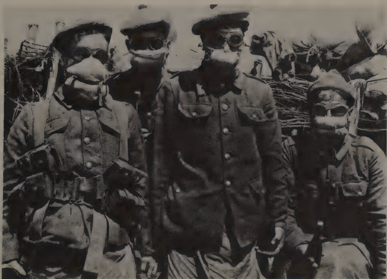
2 The first British respirators, May 1915. Each man carried a bottle of soda solution with which he was supposed to moisten the flannel. The masks were little protection: on 24 May, 3,500 men were gassed in a single four-hour attack.
