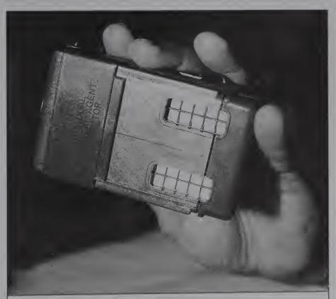
This poison gas detector could be used to tell people of an attack with a chemical warfare agent so they could take protective steps, such as wearing gas masks.
