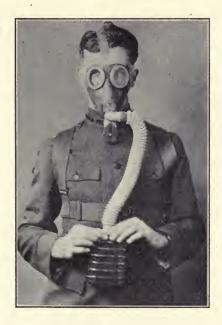
Fig. 66.—Ammonia Mask, Showing Relative Size of Canister.
