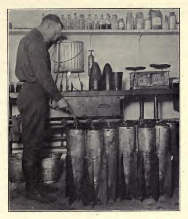
Fig. 110.—Loading Bombs with "Solid" Oil.
