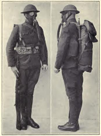
Fig. 63.—1919 Model American Mask after Adjustment.
