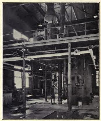
Fig. 23.—Furnace for Generating Carbon Monoxide.
