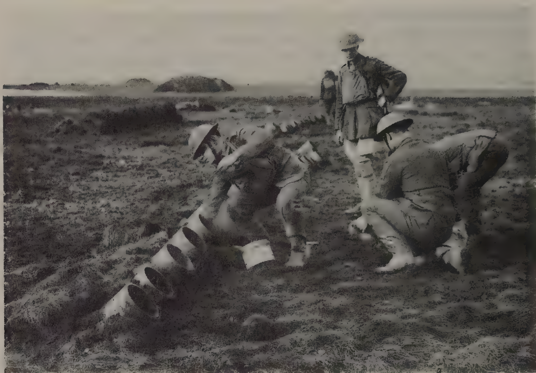
Livens projector deployed, showing placement of the propellant charges. (Courtesy of Imperial War Museum)
