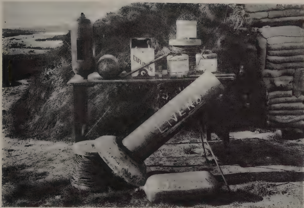
Complete Livens projector equipment—bomb, exploder, coiled leads, charges, and, in foreground, Livens projector and base-plate (propped at a forty-five-degree angle). (Courtesy of Imperial War Museum)
