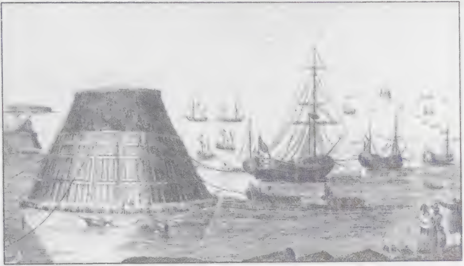
6 'View of a Cone constructed in the year 1785 being conducted to its place in the Road of Cherbourg in order to be sunk'
