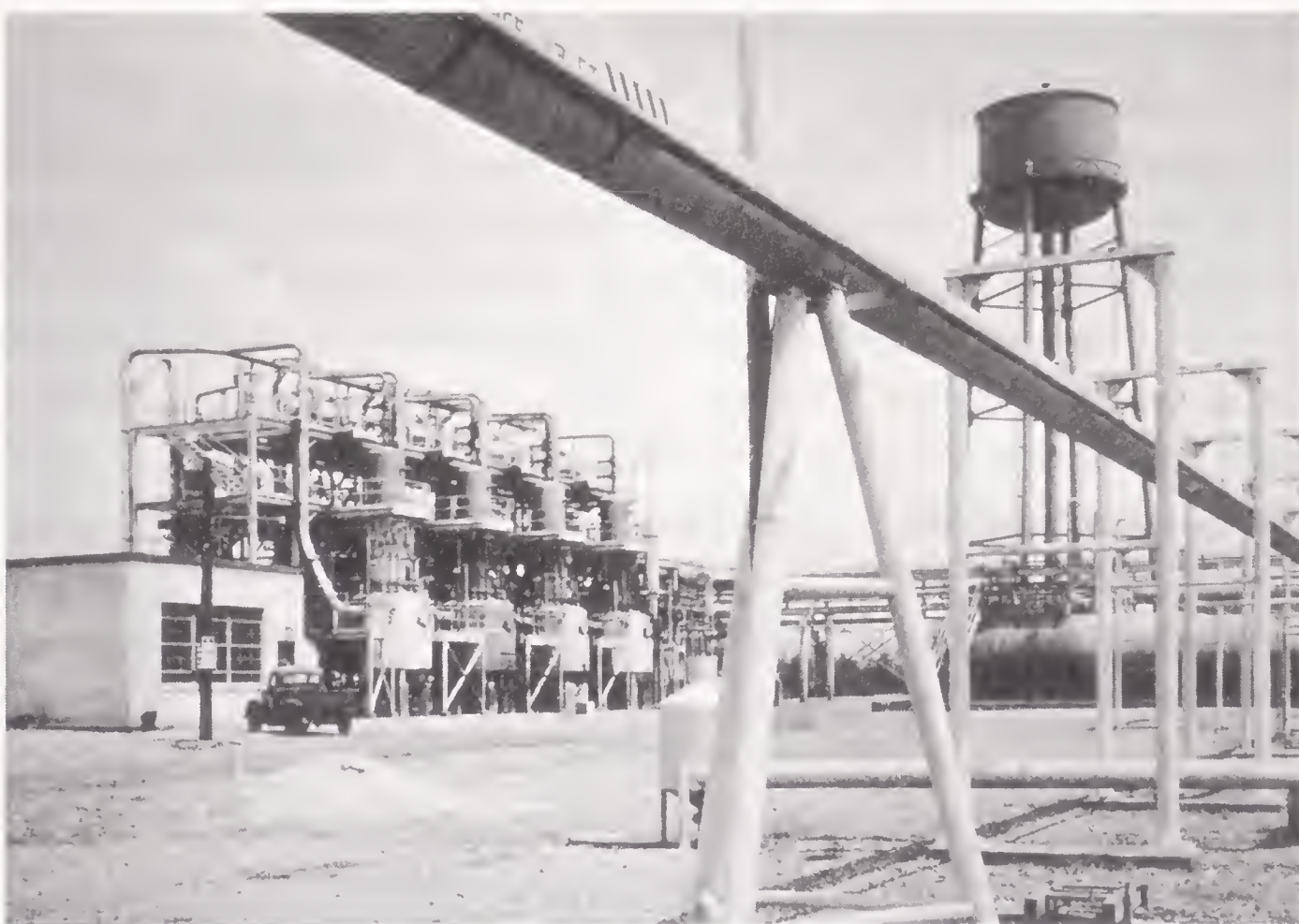
A production plant for phosphorus trichloride—the main starting material for dichlor production—in the Phosphate Development Works at Muscle Shoals.
