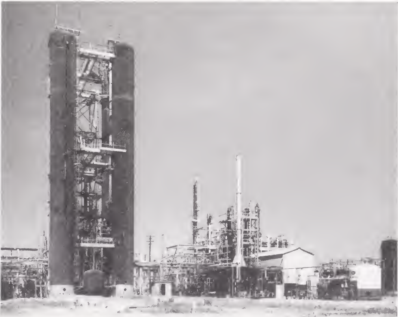
Two extraction columns from the former Dana Heavy Water Plant were incorporated into the VX production facility at Newport.
