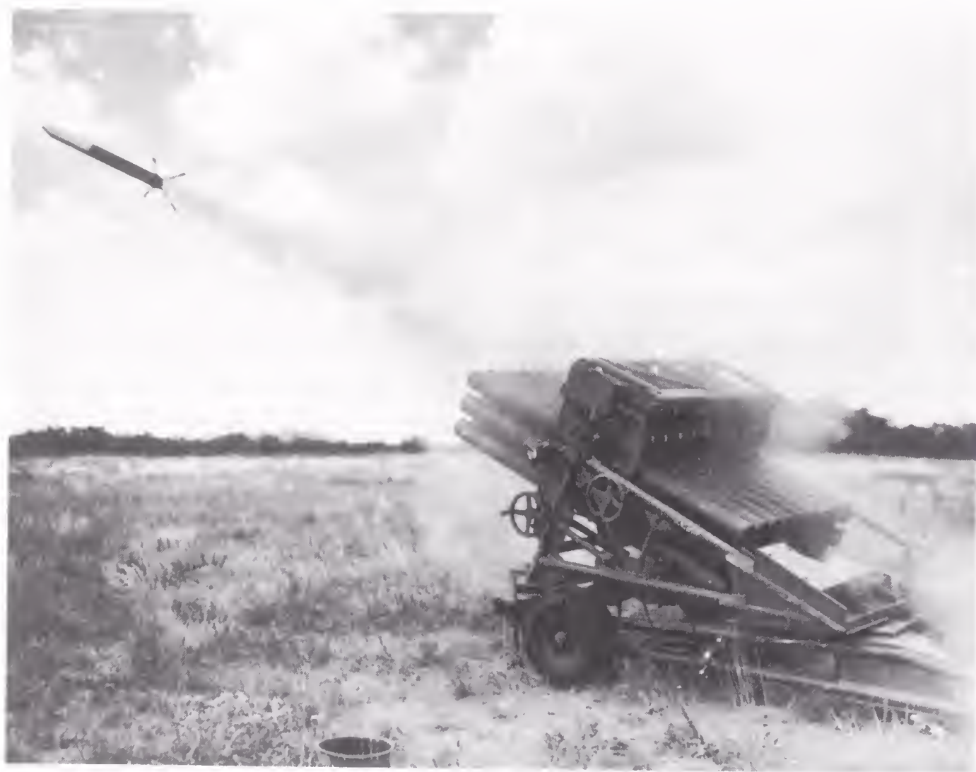
A M55 rocket with a nerve-agent warhead is test-fired from a multiple-tube launcher system. Hundreds of thousands of these rockets were produced and filled with Sarin or VX in the early 1960s. Many of the Sarin-filled rounds soon began to leak, creating a huge disposal problem for the U.S. Army.
