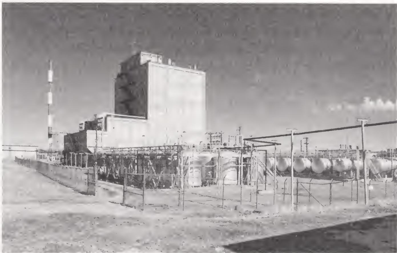
Rocky Mountain Arsenal blockhouse, which contained the final steps in the Sarin production process. The building was hermetically sealed to prevent the escape of deadly gases.
