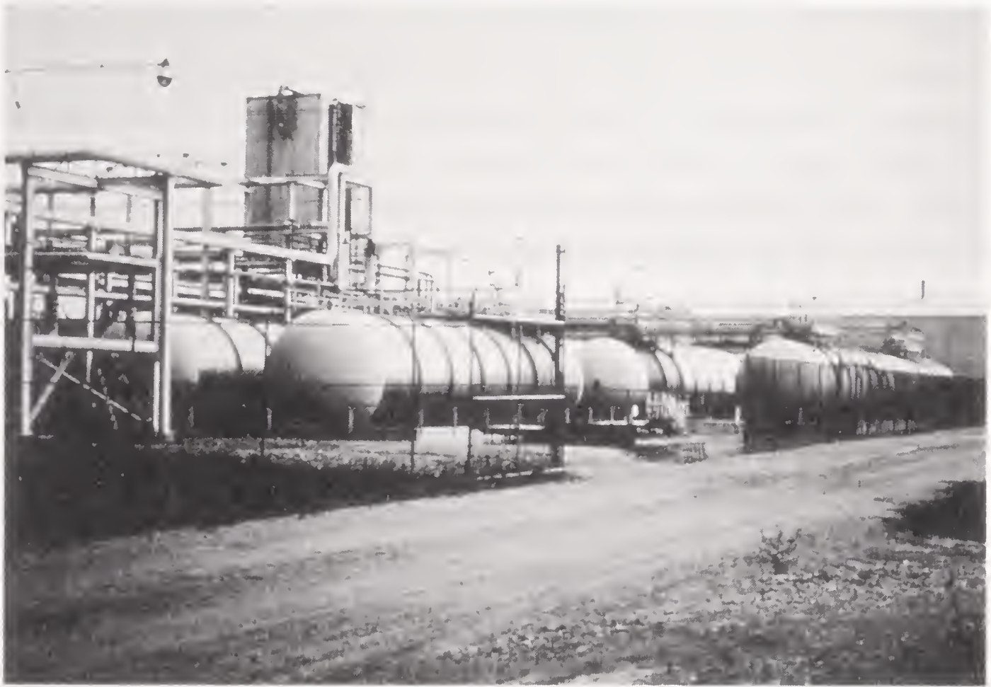
Aboveground storage tanks for bulk VX at the Newport Army Ammunition Plant. A shortage of munitions during the Vietnam War caused large amounts of bulk nerve agent to be stored on the facility grounds.
