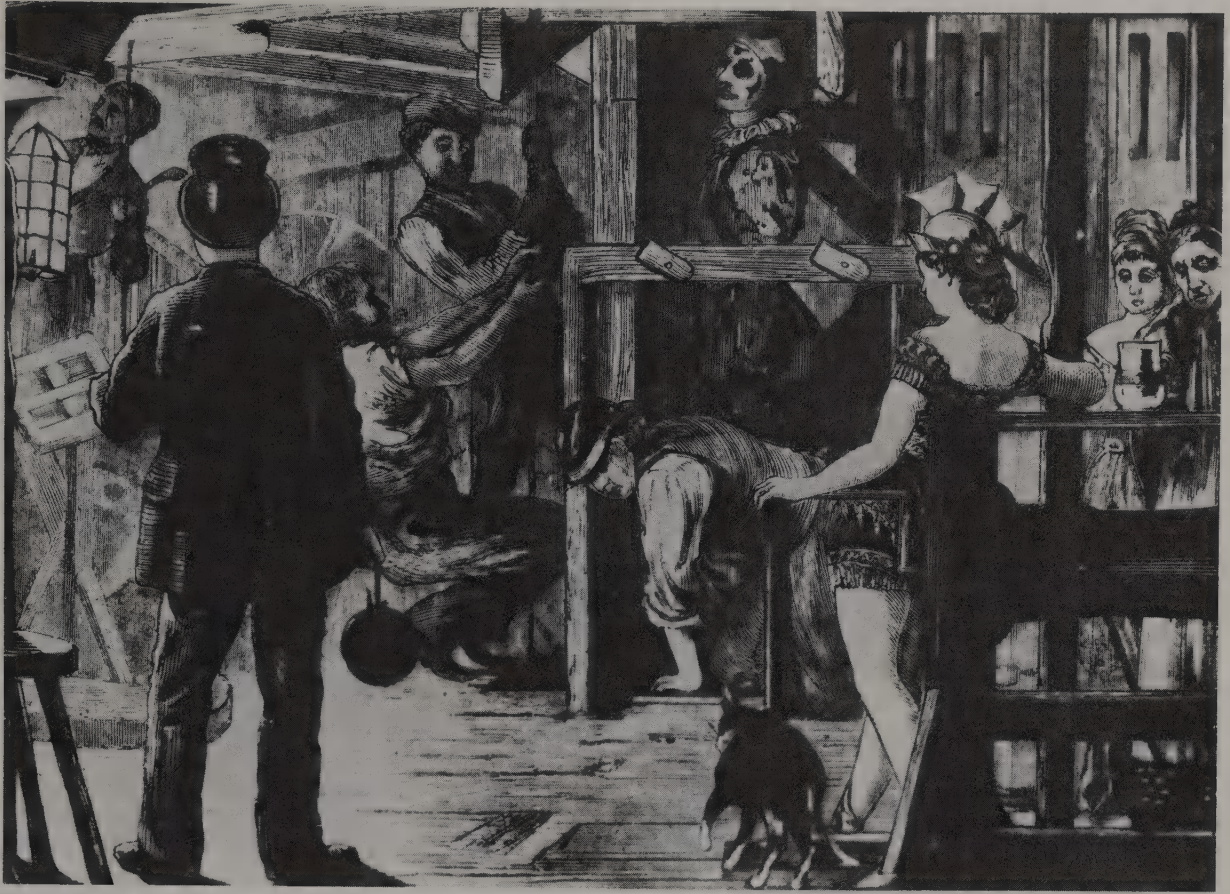
Below stage: the workings of the Star Trap. Counterweights held the platform down: when released, the performer was projected on to the stage as if by magic
