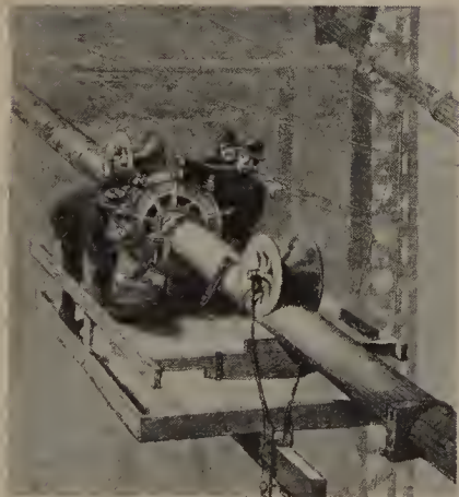
Brooklyn Bridge. Wrapping the cable
