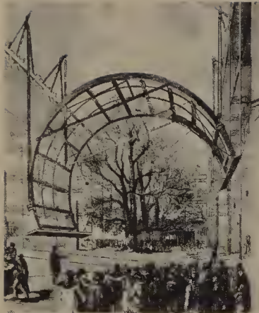
Joseph Paxton. Crystal Palace, prefabricated parts, London. 1851
