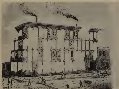
James Bogardus. Iron frame construction, U.S.A. c. 1850
