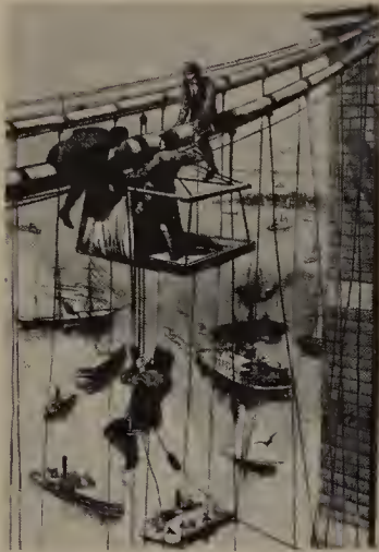
Brooklyn Bridge. Weaving steel cable
