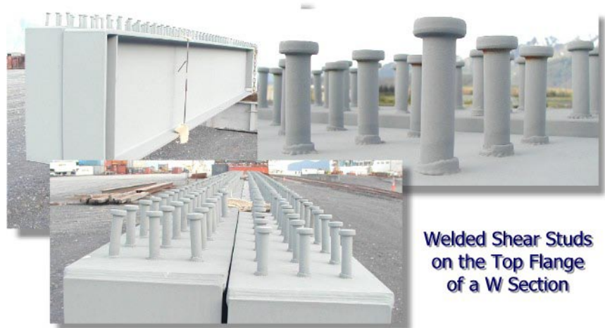
Figure 10.2.2 Typical Welded Studs
