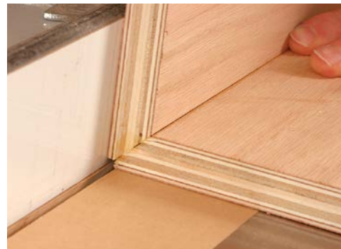
Rabbet the corner. Cut a \frac{1}{8} -in.-sq. rabbet in each corner using the tablesaw or router.
