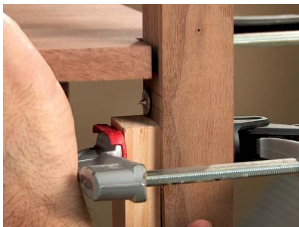
Locate the shelf. A support block clamped to the leg holds the shelf in place.
