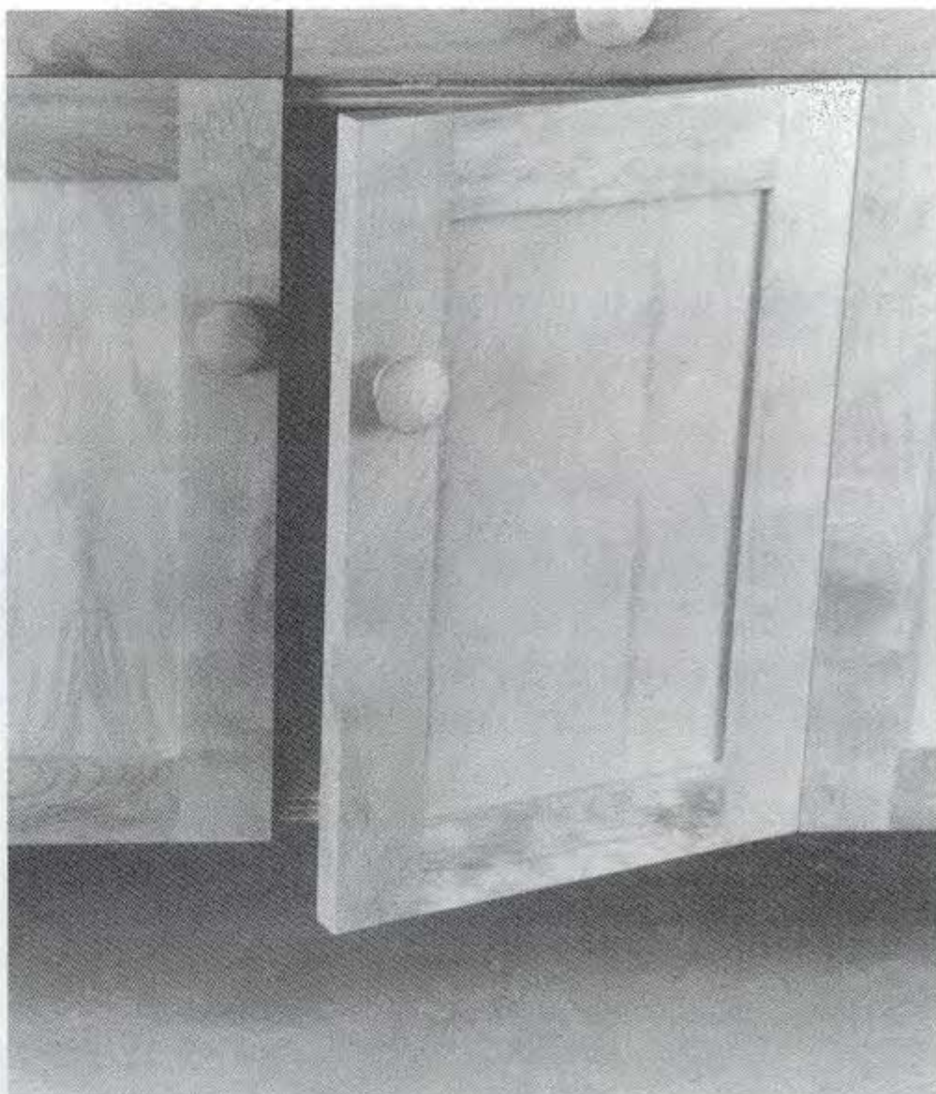
1-16 Traditional frame-and-panel construction , such as these cabinet doors, employs floating joints. The panels expand and contract in grooves cut in the inside edges of the rails and stiles.
