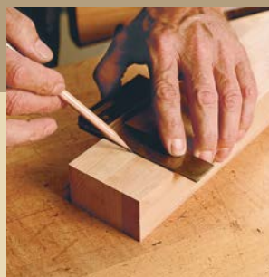
MARK THE SHOULDER LINE. All pieces cut by hand must be marked on every side and end.
