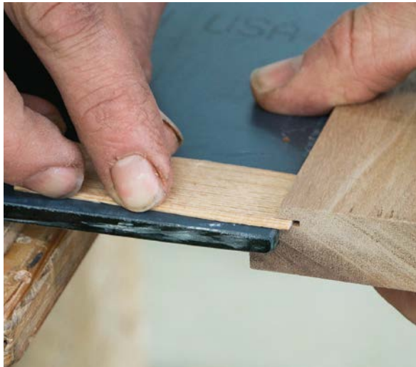
A 1/16-in. shim holds the mirror in place.
