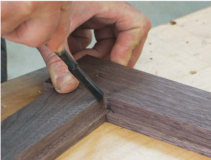
Use a chisel to square off the end of the stopped rabbets.
