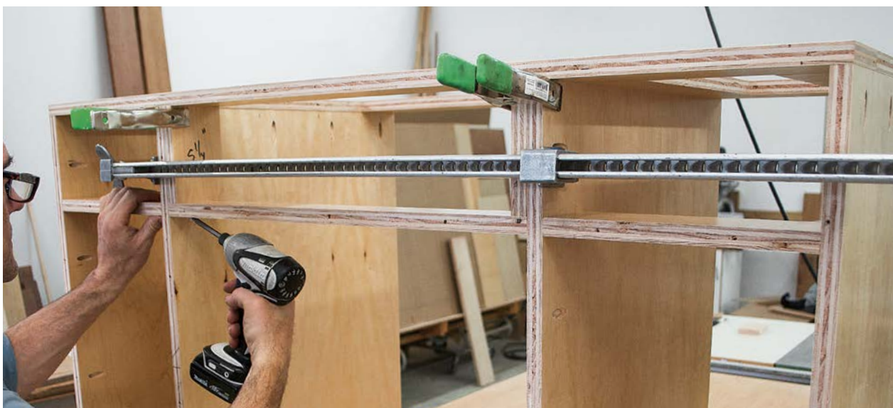
Use the 5½-in. plywood scraps to help locate and install the under-sink partition.
