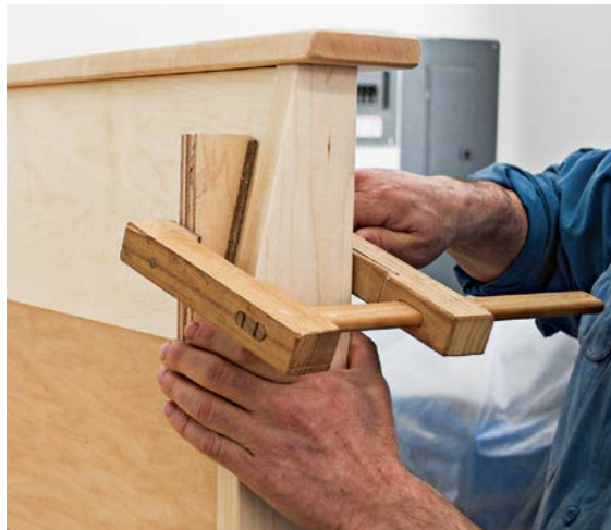
Apply glue to the biscuit holes in the furring strips and plywood panel.
