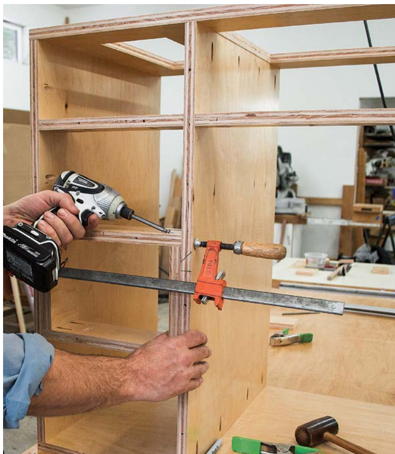
Install the middle drawer partition on the left-hand side last, again using plywood scraps to locate and install the partition.
