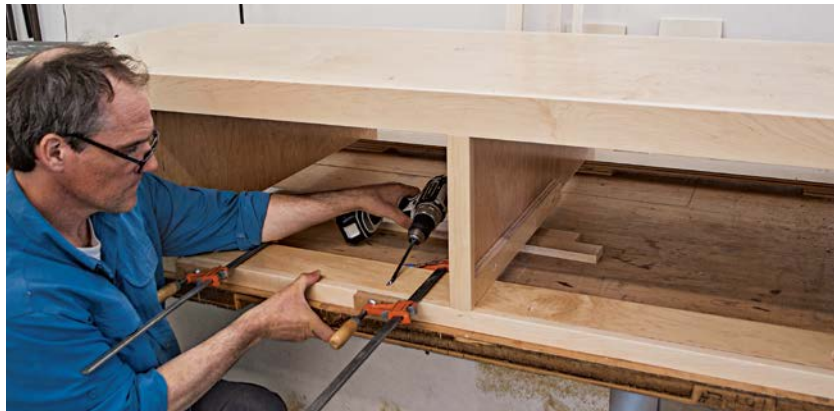
Attach the bottom face frame rail first, using clamps wherever there is a screw to hold it in place.
