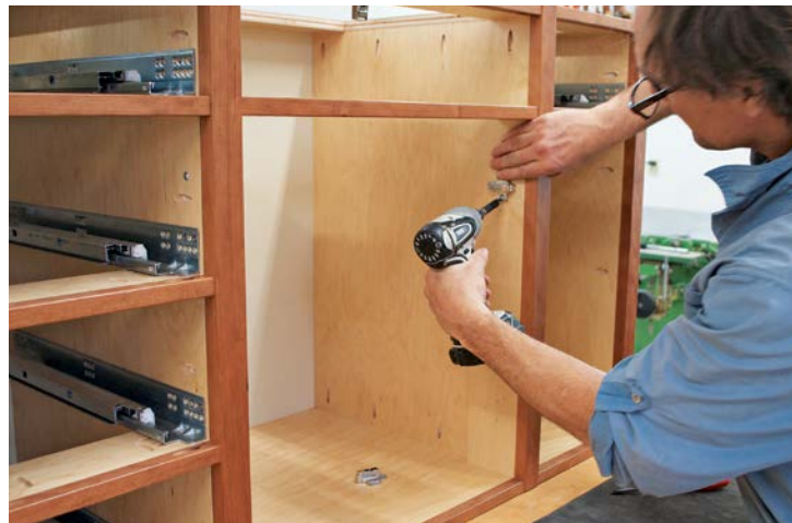
A strip of plywood is needed to bring the hinges out far enough to reach around the face frame. Attach the hinge bases to the strip with screws.
