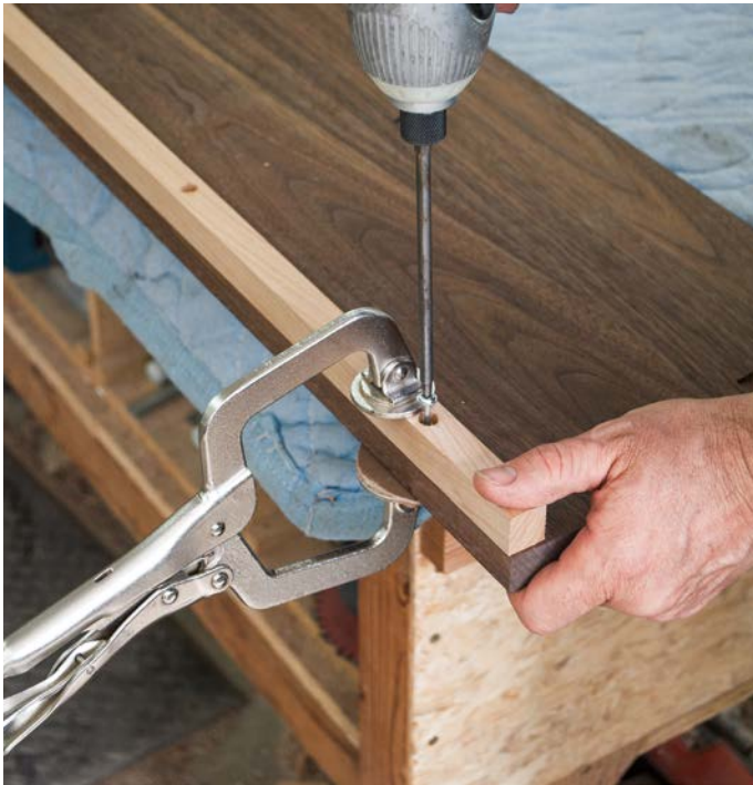
Add the support strips to the inside of the mattress rails with countersunk pocket screws.
