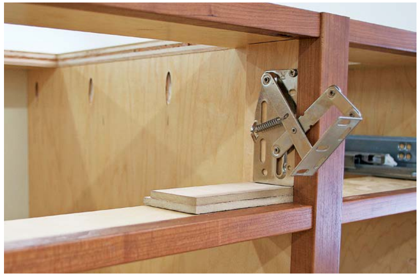
Install the hinges for the tip-out tray on both sides of the under-sink opening.
