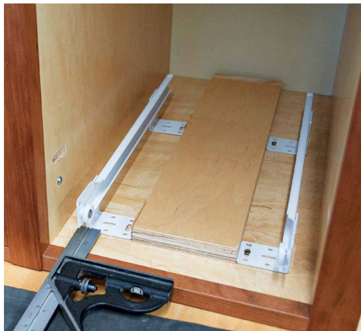
When installing the hardware for the pull-out garbage container, use a scrap of plywood to make sure that the runners are mounted parallel.
