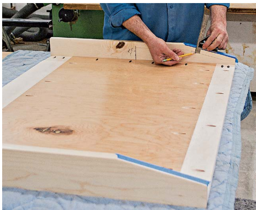
Use a try square set at \frac{7}{8} in. to mark the locations of the furring strips on the inside face of the corner posts.
