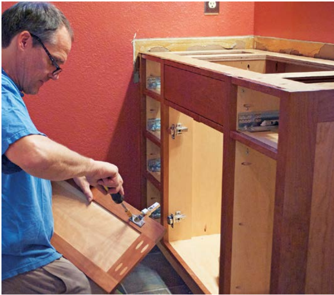
Attach the Euro hinges to the doors using a Phillips screwdriver to adjust the hinges for a perfect fit.
