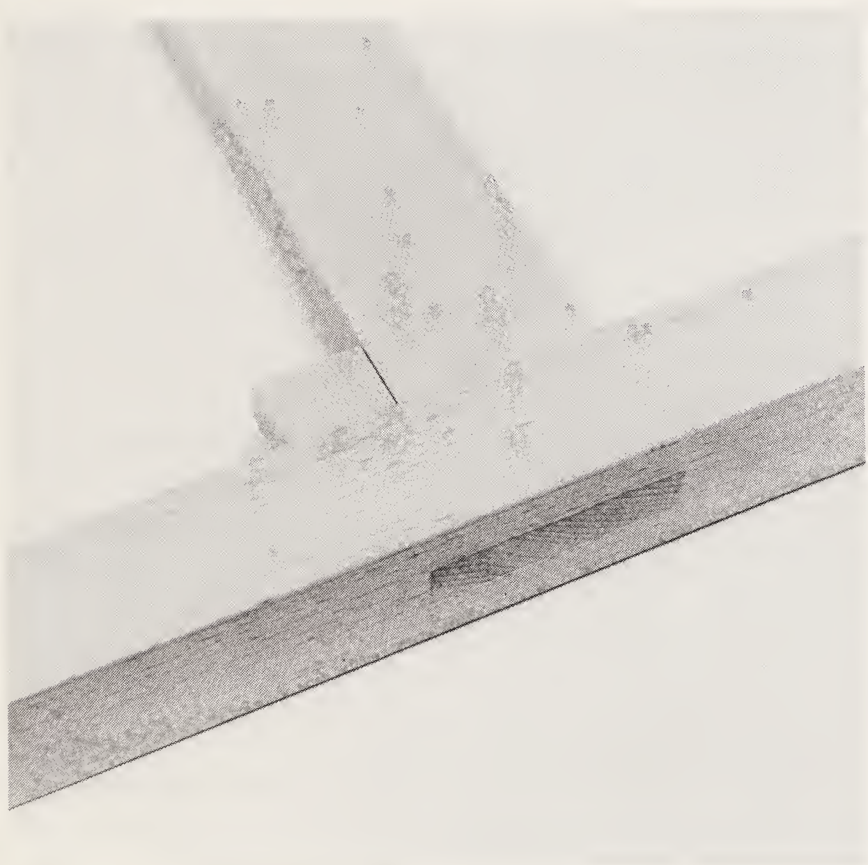
Figure 3 Sage-kama ( wedged through half dovetail )
