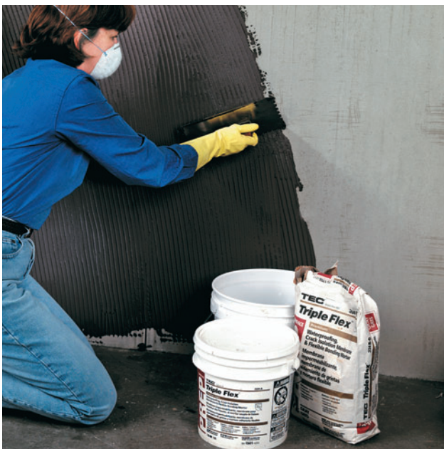
Waterproofing/isolation membranes are an easy way to add waterproofing and crack protection to existing walls. This application is especially suited to smooth, solid concrete surfaces. The tile adhesive is applied directly to the membrane after it dries.
