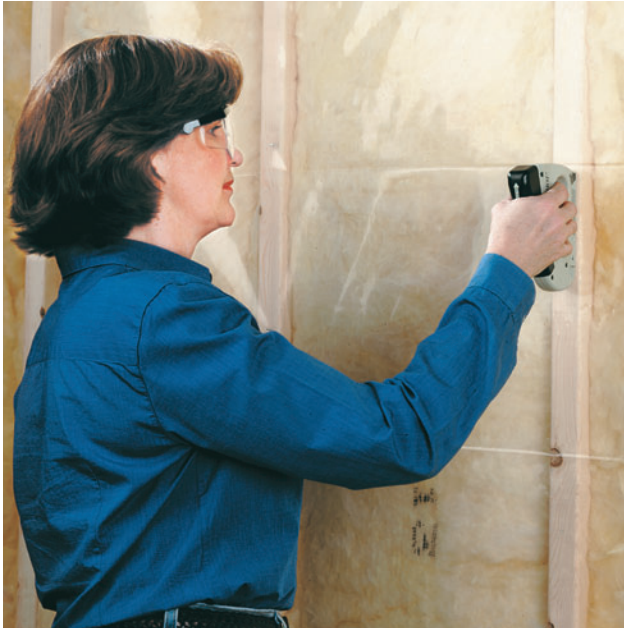
A water barrier of 4-mil plastic sheeting can be stapled to studs before installing cementboard or fiber-cement board.
