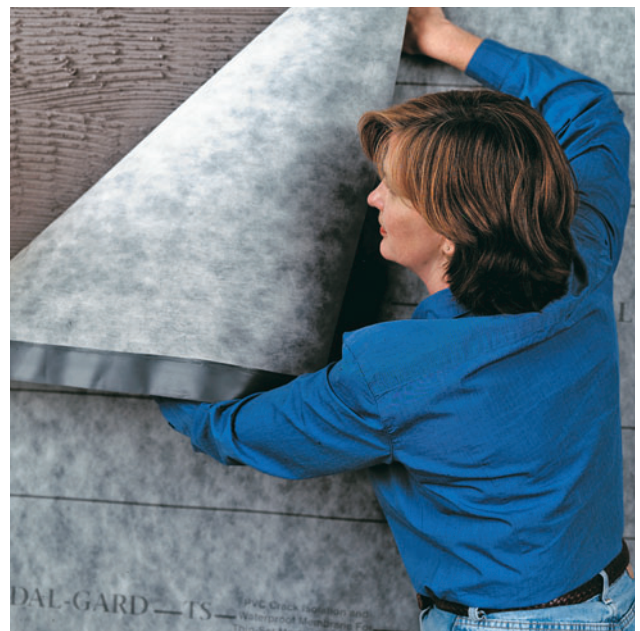
Isolation membrane may be used on wall and ceiling surfaces in areas such as steam rooms and saunas that have extreme temperature fluctuation and high humidity. The membrane is typically installed with mortar, but some membranes must be used with a specific bonding agent.
