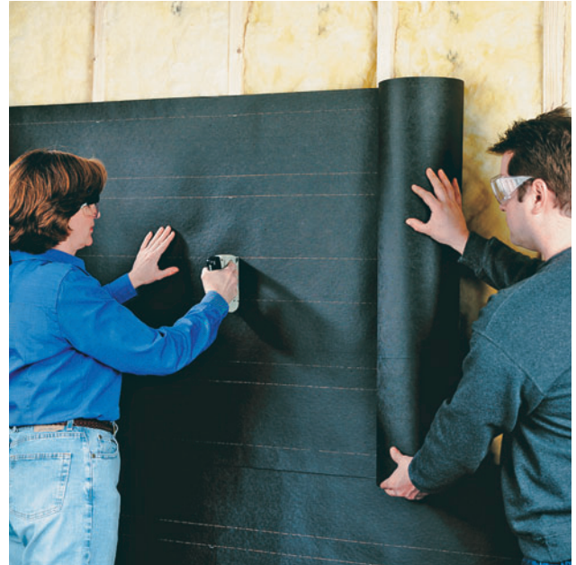
Building paper (15#) can also be used as a water barrier behind cementboard and fiber-cement board. Start from the bottom and install horizontally so each layer overlaps the previous one by two inches.
