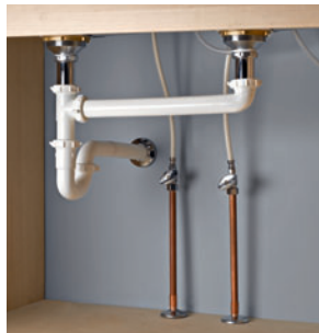
20 Connecting a Kitchen Drain . . . . . 84
