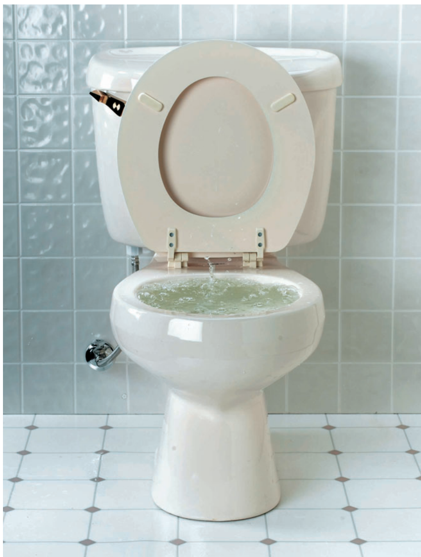
A blockage in the toilet bowl leaves flush water from the tank nowhere to go but on the floor.
