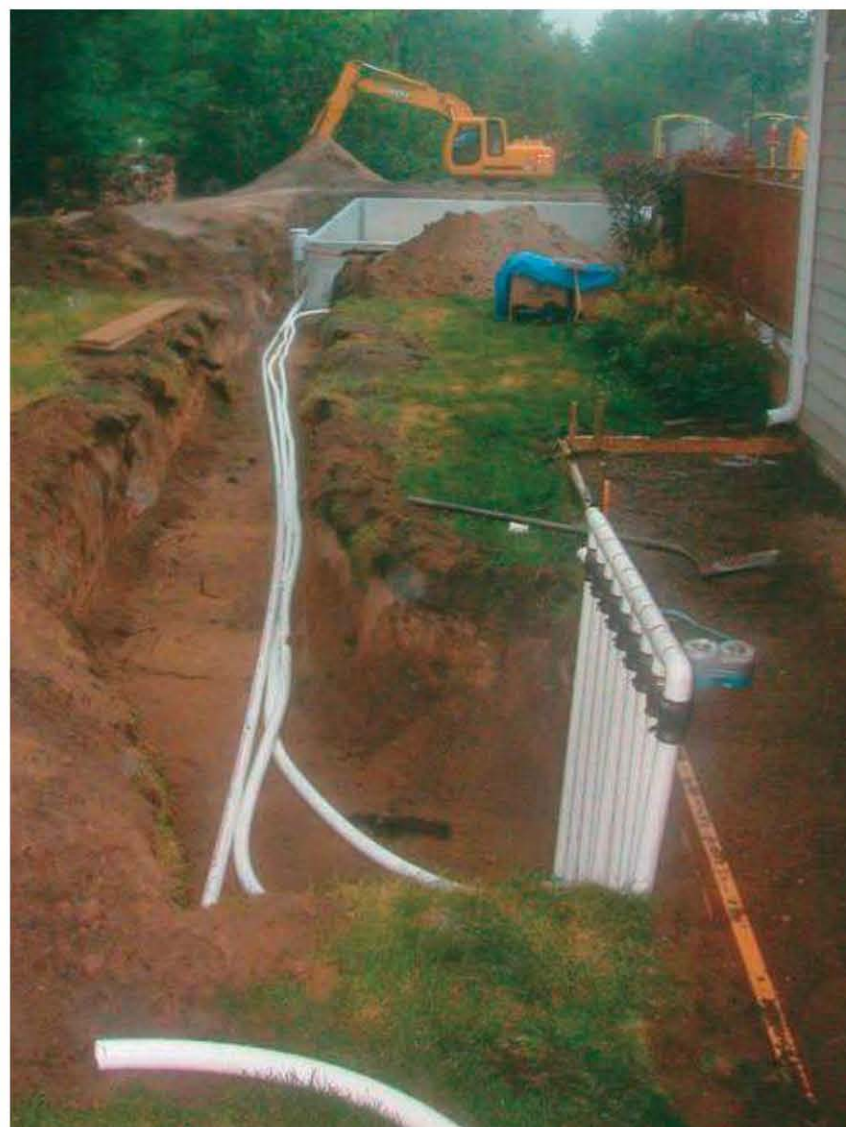
Underground plumbing lines are run from the pool drain and skimmer locations to the intended location of the equipment set.
