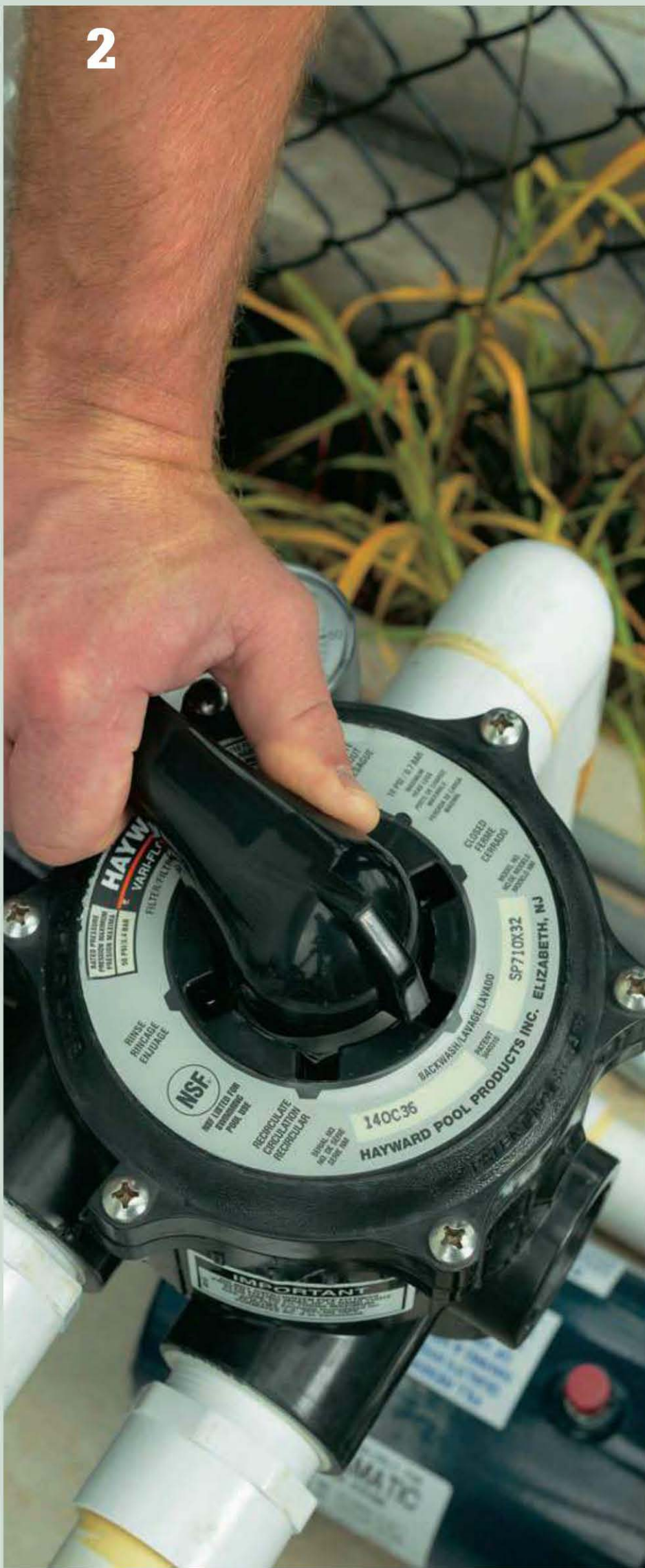
Turn the handle on the backwash valve (a multiport valve) from the "filter" setting to the "backwash" setting.
