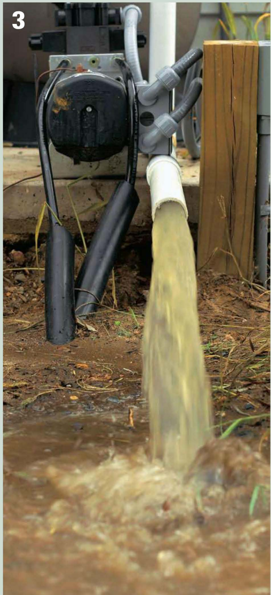
Let the water discharge. You may want to attach a piece of piping or a flexible tube to the discharge outlet to direct water away from the equipment set area. Restore power to the pump. Let the pump run for about 90 seconds. Shut off power to the pump and change the valve setting to "rinse." Restore power to the pump and run at "rinse" for 10 to 15 seconds. Shut off power, set valve back to "filter" and restore power to resume normal operation. The process normally results in the loss of up to 100 gallons of pool water, so it may be necessary to add water to the pool.
