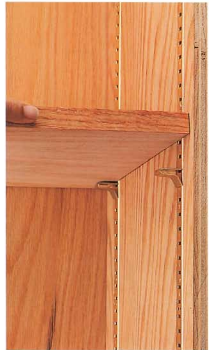
C. Insert a metal shelf clip into each standard, and place a shelf on top of each set of clips.
