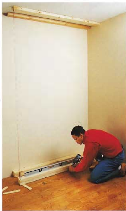
B. Use a plumb bob suspended from the outside corners of the top plates to align the sole plates. Anchor the plates with 3" screws driven toenail-style into the floor.
