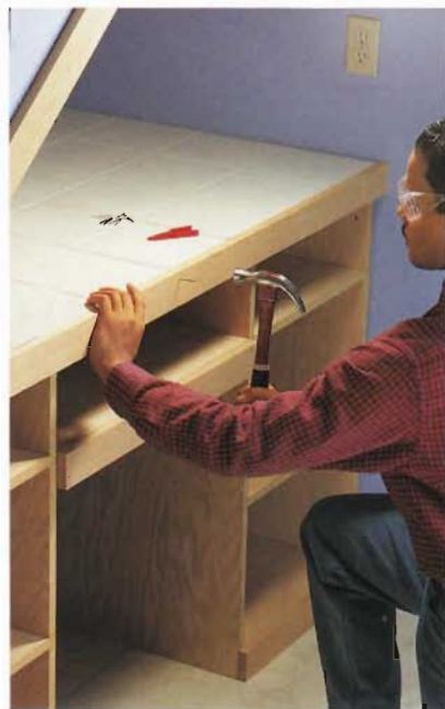
J. Attach the countertop rail with 2" finish nails driven through pilot holes.
