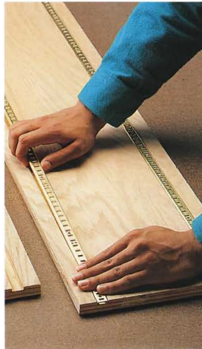
B. Test-fit the standards in the dado grooves, then remove them.
