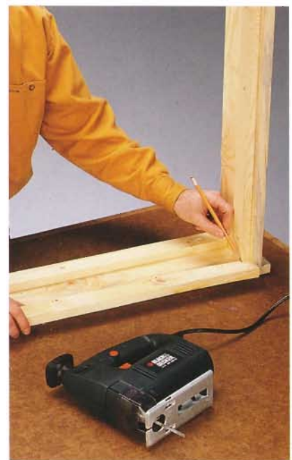
C. Attach the cleats to the inside face of the box front, trimming them if necessary.
