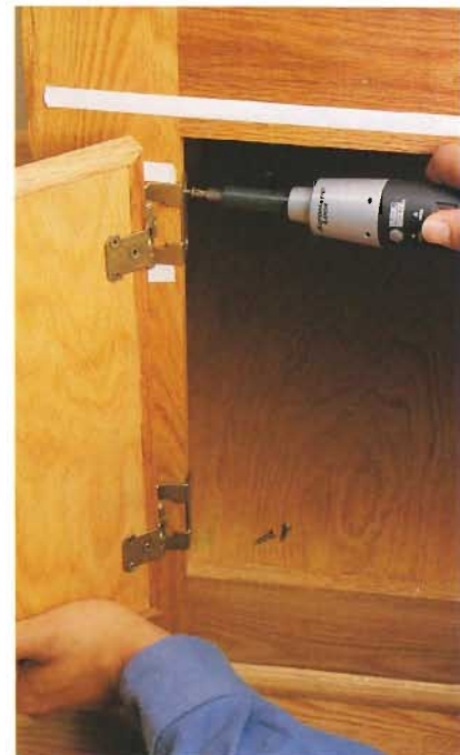
C. Install the door by driving the mounting screws into the edge of the cabinet frame.
