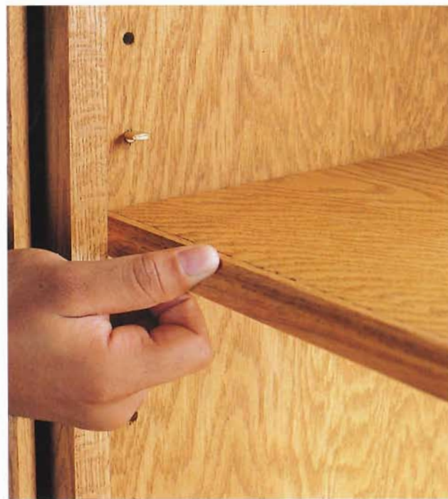
B. Build shelves that are \frac{1}{8} " shorter than the distance between the risers, and install them with four \frac{1}{4} " pin-style shelf supports.
