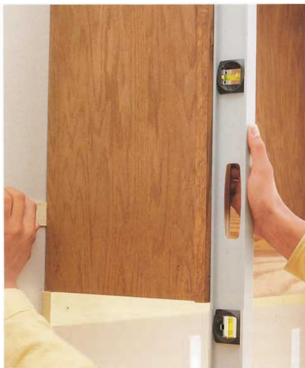
H. Check to make sure the cabinet is plumb, shimming behind the cabinet if necessary.
