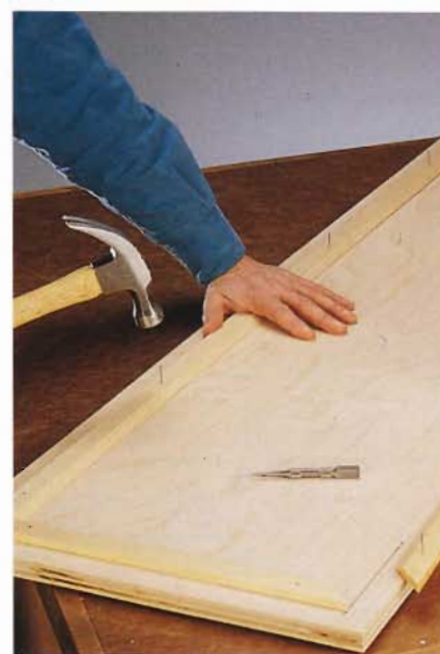
C. Attach the stop molding to the door, 1" in from the top, bottom, and side edges.
